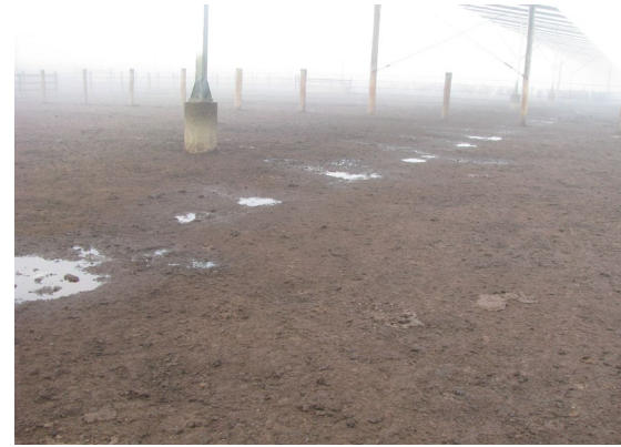
Corrugated iron sheets can concentrate rainfall runoff to localised areas; ponding will damage the pen surface.
