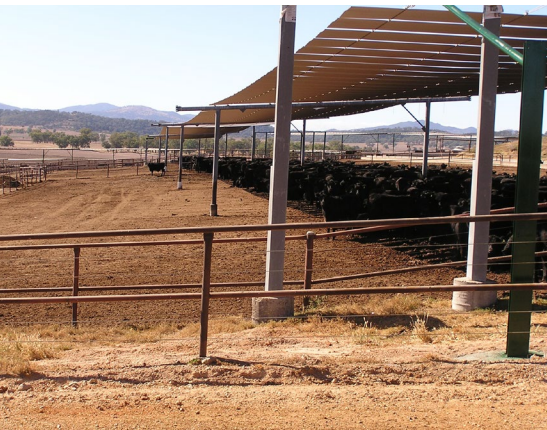
Clear-span structures minimise columns within the pens. Columns are best positioned in the subdivision fence lines.
