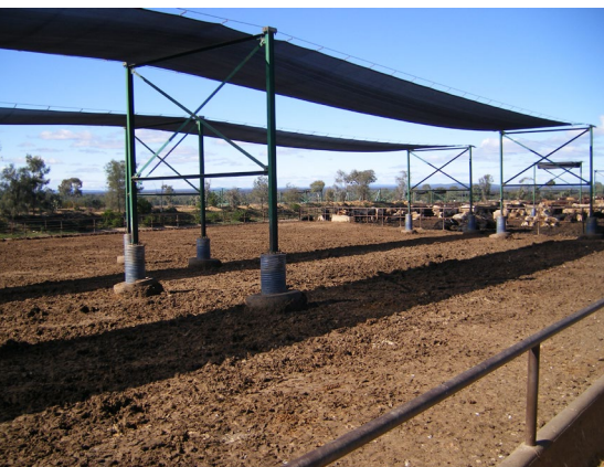
Too many support posts make pen cleaning more complicated; fewer structures would need to be strengthened. Encasing posts in concrete protects them from corrosion, damage during pen cleaning and reduces injury to cattle.
