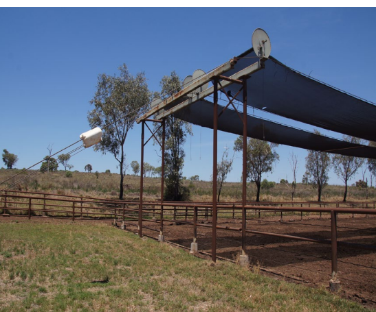
This shade can be retracted using a pulley system connected to the PTO shaft of a tractor.
