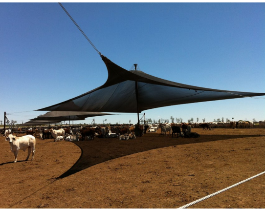
A taut peaked shade cloth structure. Sloping fabric will ensure good shedding of water and hail.
