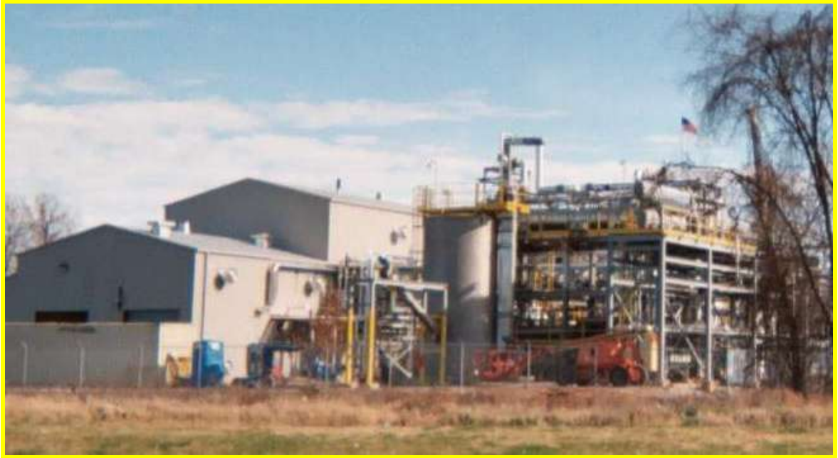
Figure 4.10: Photo of the CWT TDP Plant
