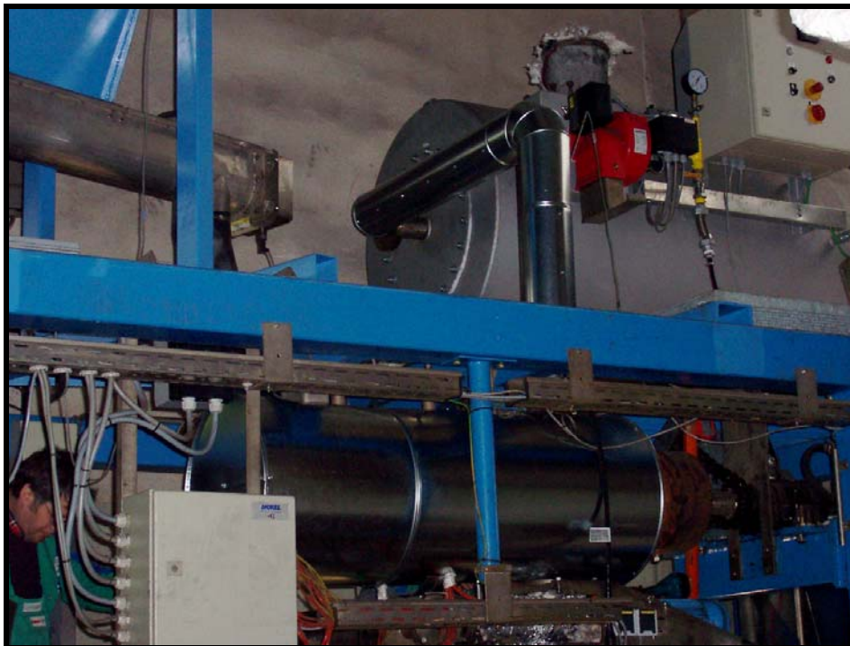
Figure 4.23: ZWT Pyrolysis Pilot Plant
