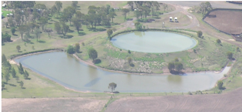
Photograph 14 – Turkey’s nest water storage
