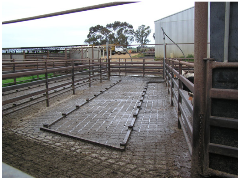
Photograph 8 – Interior of a feedlot cattle wash showing ground mounted belly sprays
