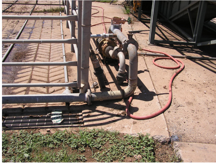
Photograph 9 – Flooring, pipe work and drain of a feedlot cattle wash
