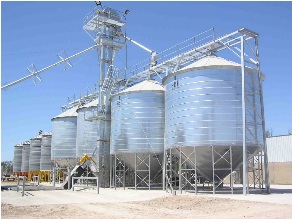
Photograph 1 - Typical grain storage system
