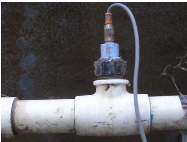
Photograph 36 – Installed water meter M6 at Feedlot E
