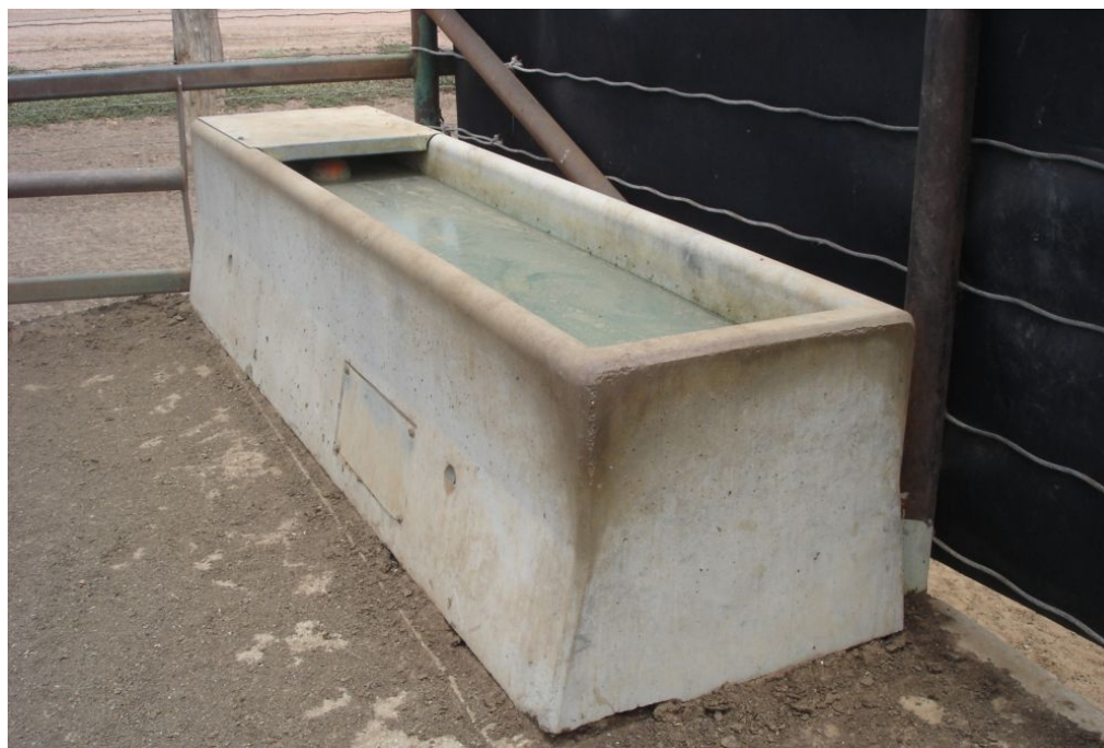
Photograph 49 – Small 3-m trough type showing steel float cover (Feedlot A)
