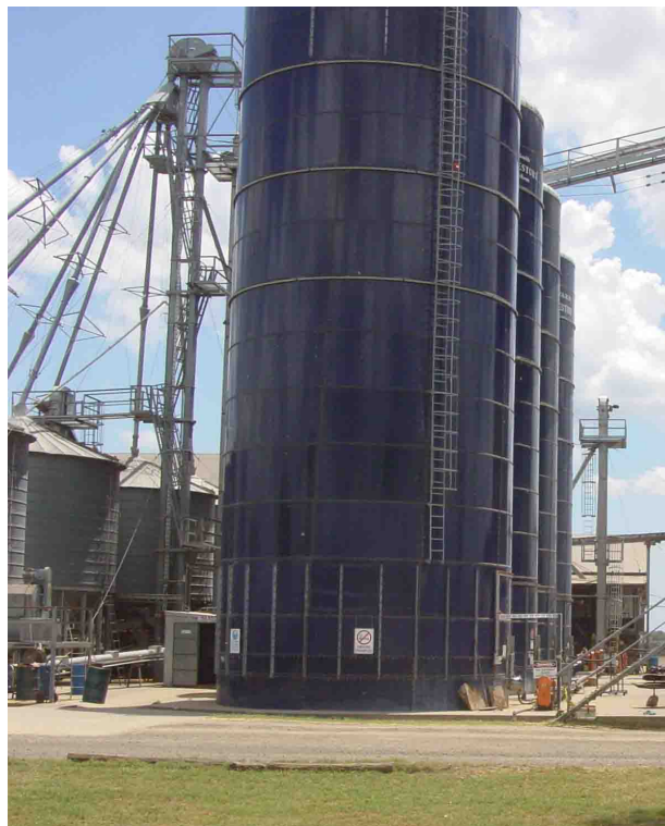
Photograph 5 – Typical reconstitution silos
