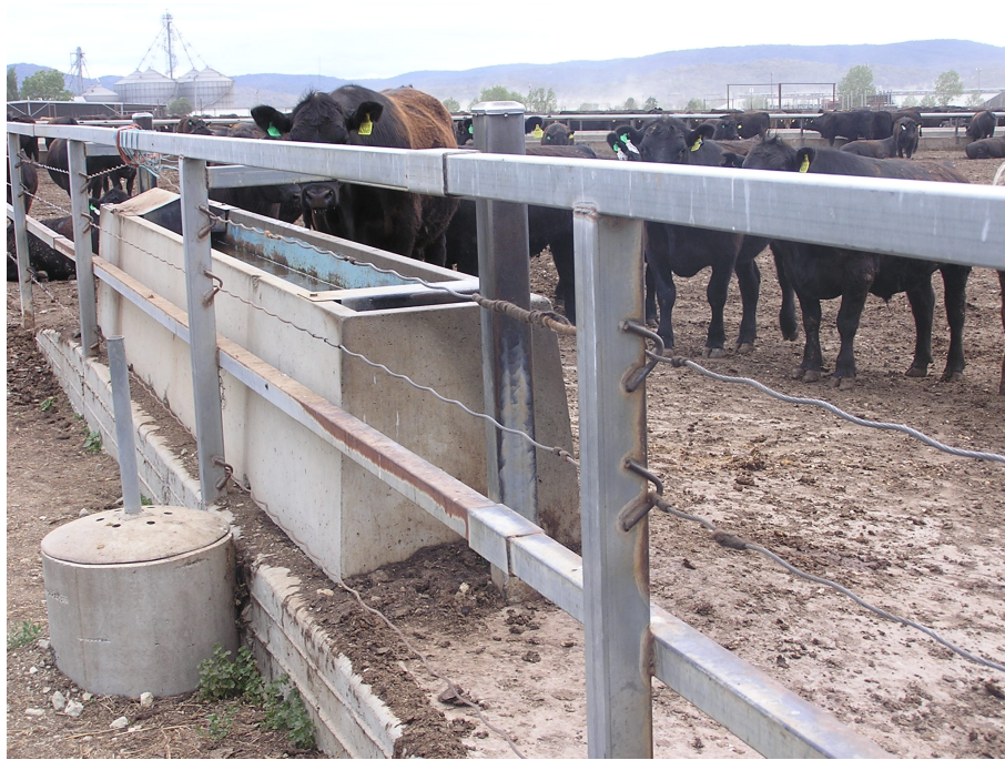
Photograph 60 – Standard large Type-2 trough with trapezoidal cross-section (Feedlot F)
