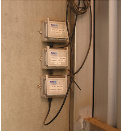
Photograph 35 – Installed water meter M9 at Feedlot C
