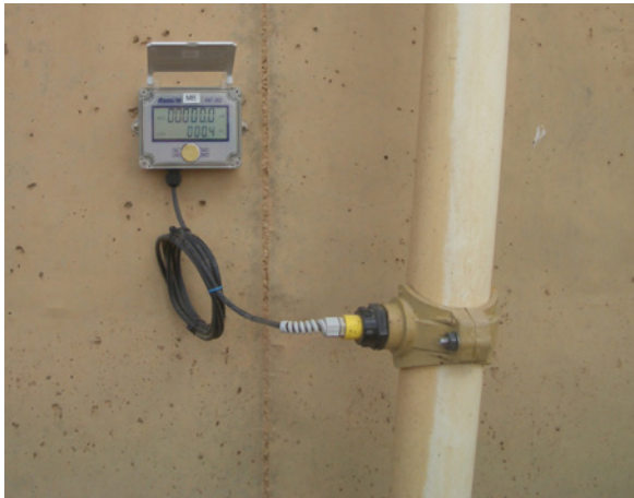
Photograph 29 – Installed water meter M8 at Feedlot B
