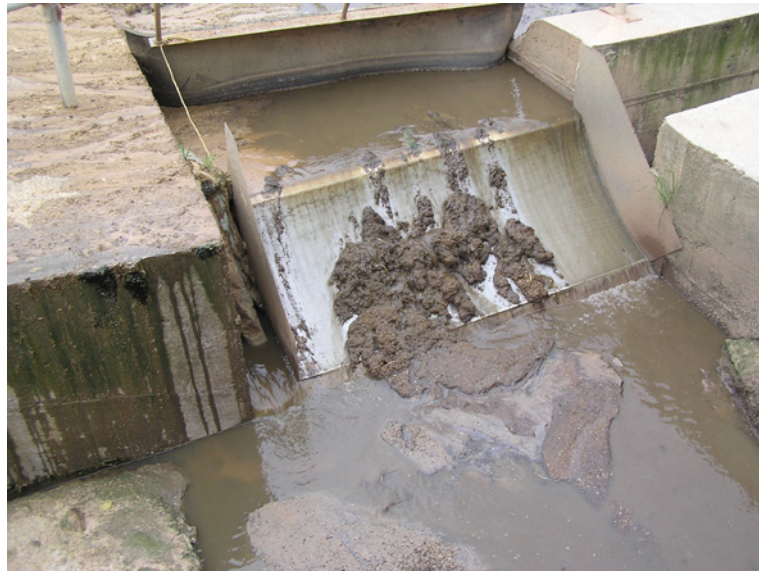
Photograph 11 – Cattle wash wastewater sump
