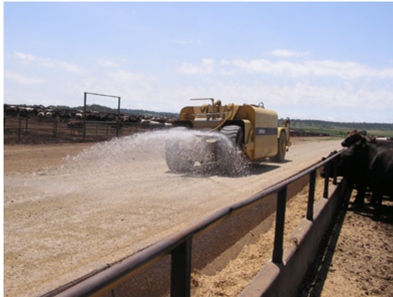
Photograph 16 – Dust suppression using a water tanker
