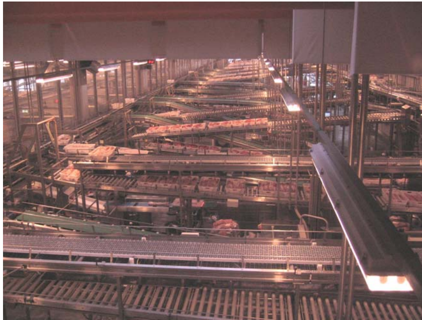
Part of the conveyor system at Danish Crown, Horsens, Denmark.
