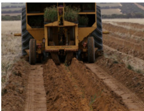
Tree planter demonstrating pressing root ball into the soil to reduce risk of air pockets that prevent root growth
