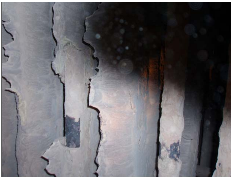
Figure 4.13: Example of Ash Fusion on Boiler Tubes
