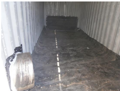
Fig 3: Empty space in lower container with con-condensables inlet (left) and By-products building inlet (far end) with air flap.
