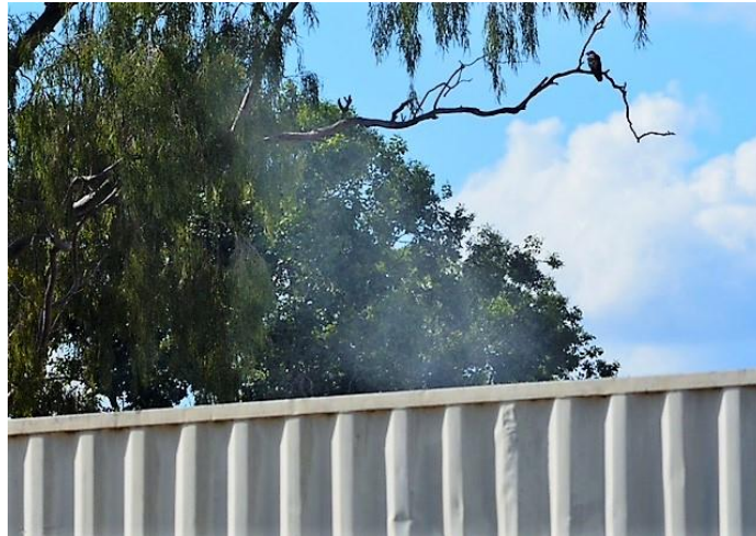
Fig 32: Water Vapour Plume due to Short-Circuiting within the Media
