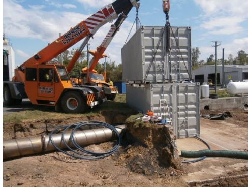
Fig 1: Shipping Containers being placed on-site
