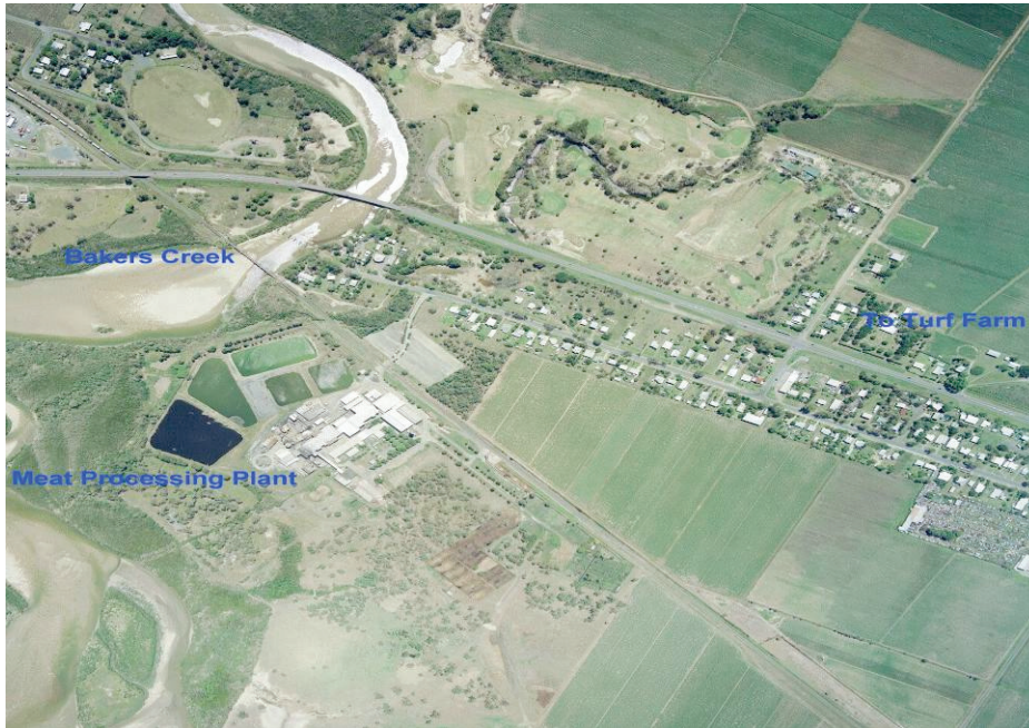
Aerial photograph of the Borthwicks plant and Bakers Creek area.
