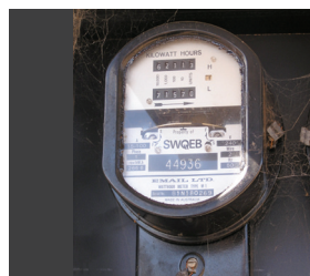
Figure 2: Electromechanical induction meter
