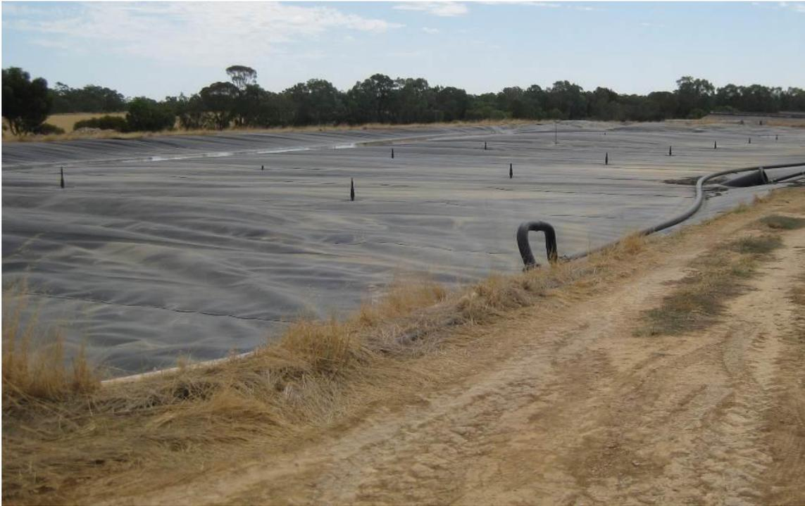
**Photograph 65 – Covered anaerobic pond (CAP)**
