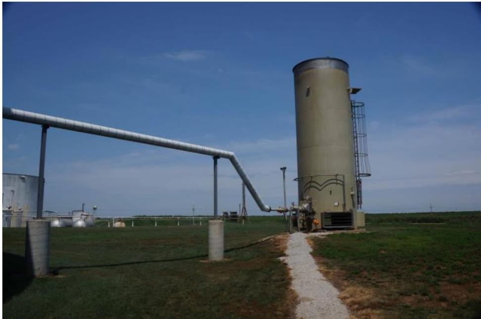
**Photograph 36 – Excess biogas flare**
