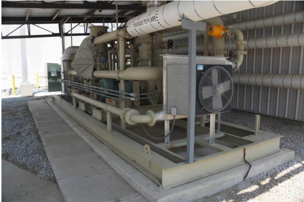
**Photograph 35 – Biogas pump from digester to ethanol plant**
