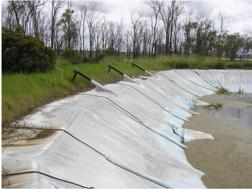
**Photograph 68 – Sludge extraction pipelines (deflated pond cover)**
