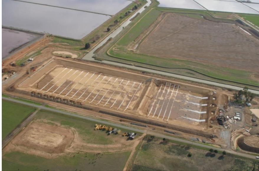
**Photograph 66 – Installation of sludge removal pipe system**
