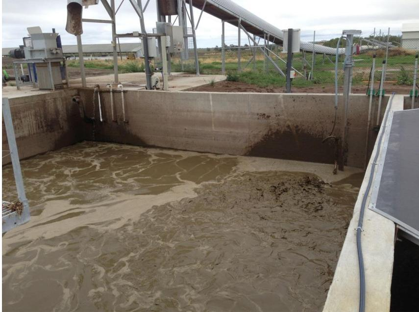
**Photograph 61 – Mixing tank with delivery of manure by conveyor**
