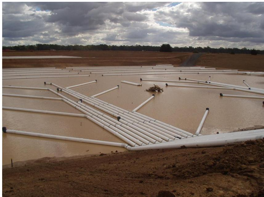
**Photograph 67 – Installation of sludge removal pipe system**
