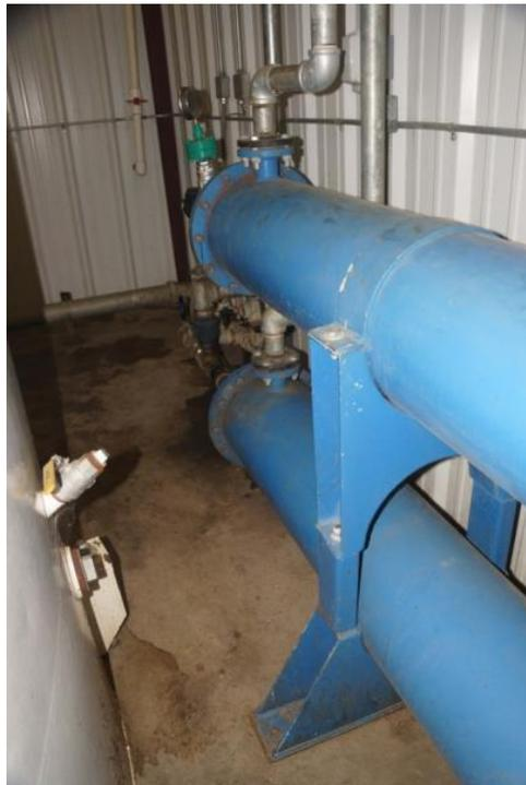
**Photograph 22 – Heat exchanger on influent line**
