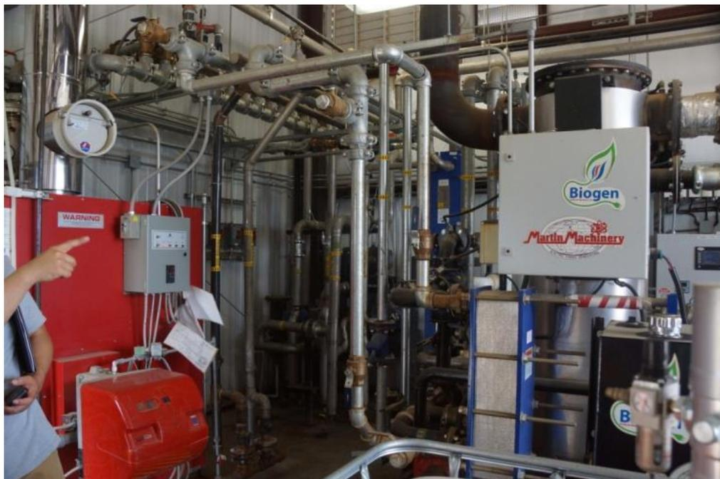
Photograph 26 – Control system for anaerobic digester and generator
