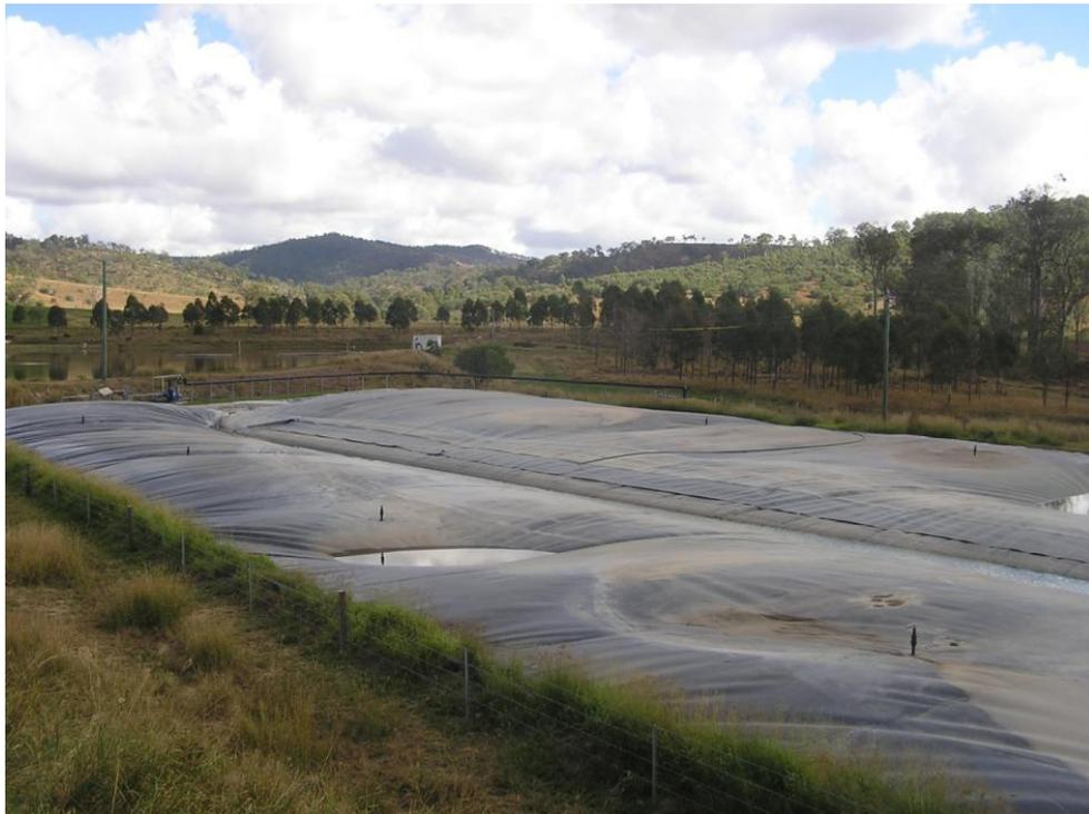
**Photograph 17 – Covered anaerobic pond for biogas production**
