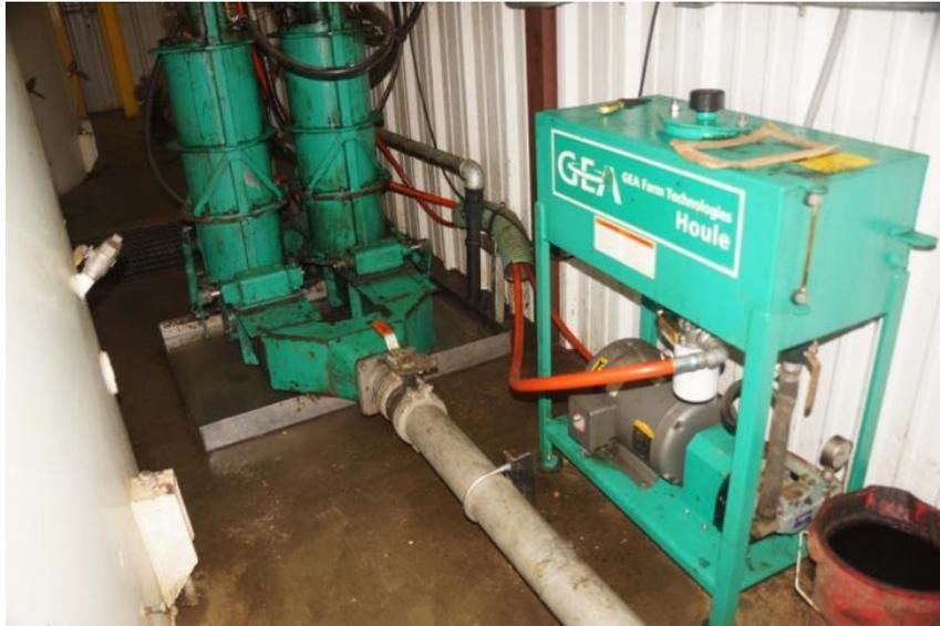
**Photograph 23 – Positive displacement pumps on influent line**
