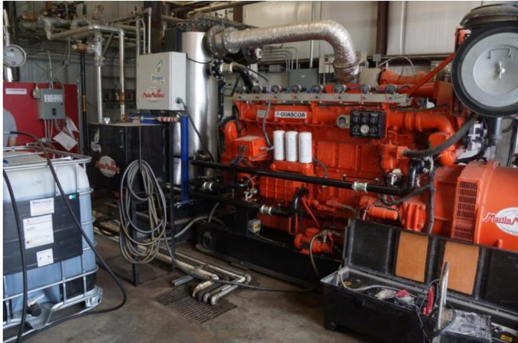
Photograph 25 – Electricity generator using biogas
