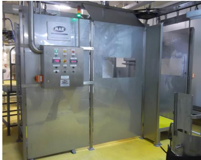
Fig.9 Installation progress images
