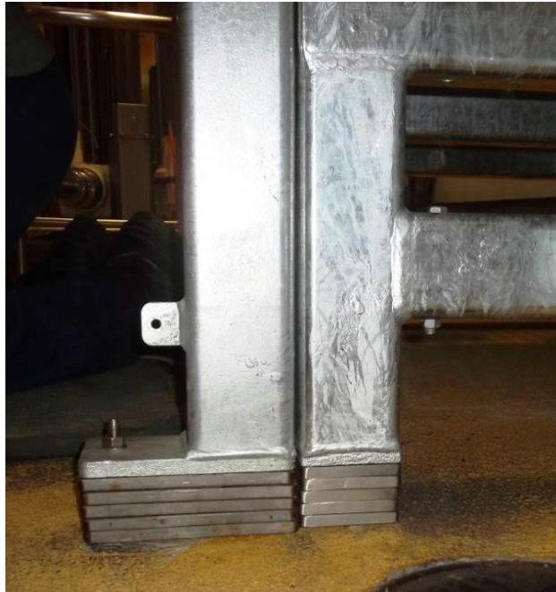
Fig.11 Packers required under robot base feet
