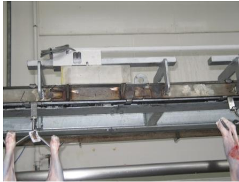
Photo 1. Load cell fitted into the overhead rail
