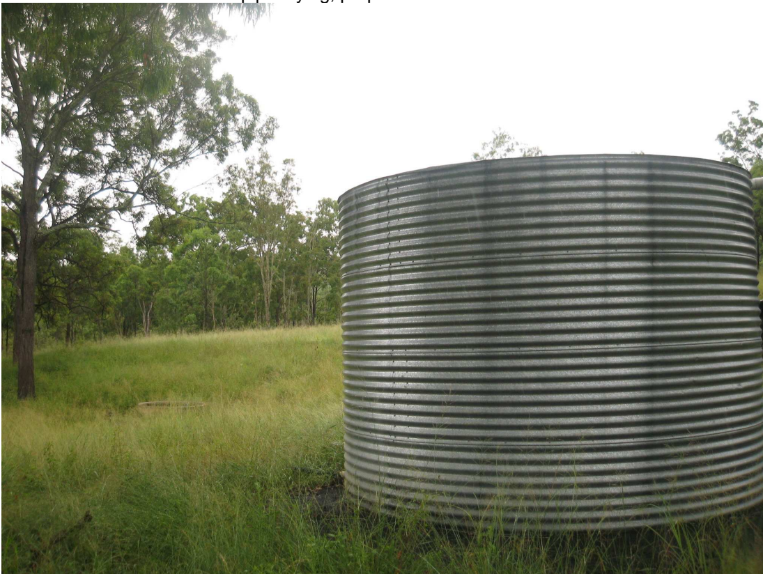
Tank installation and trough in background to the left of tank.
