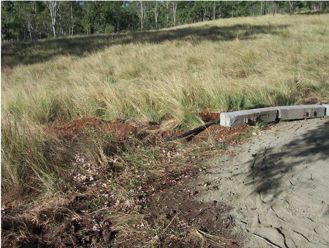
After pipe laying, preparation for tank location
