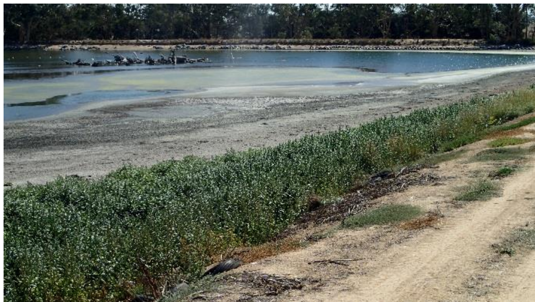
Photo 5: Aerobic Pond Sludge towards pumped outlet
