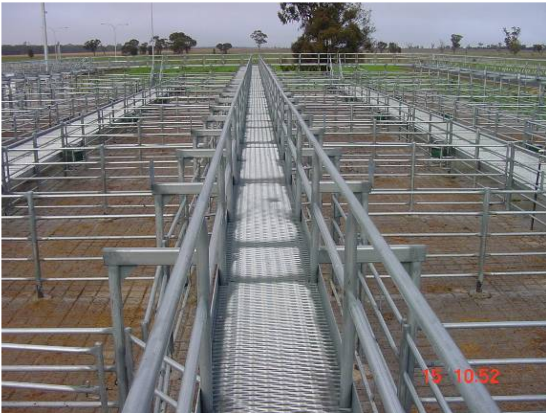
Photograph 1 – Concrete floor in a saleyard
