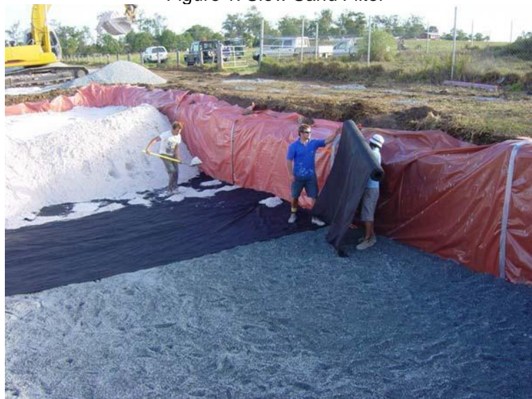
Figure 1: Slow Sand Filter
