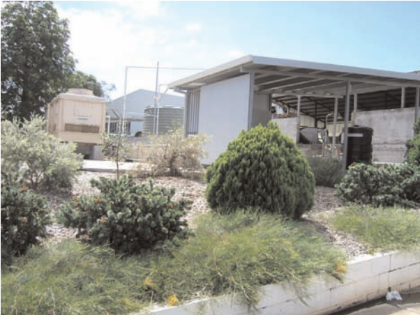
The water reuse plant with coolboys at the left rear
