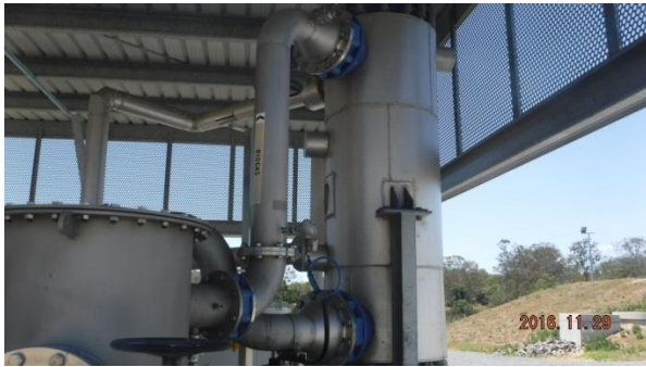
Figure 13. Biogas chiller
