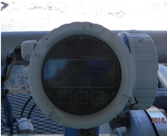
Figure 18. Biogas Flowmeter
