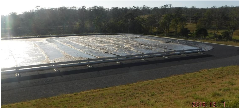
Figure 20. Biolac BNR lagoon showing air header pipe (foreground) and floating headers
