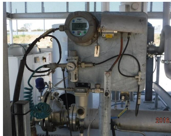
Figure 19. Biogas Methane Analyser
