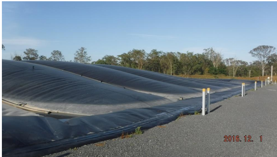
Figure 10. New CAL at the Teys Aust. Beenleigh WWTP
