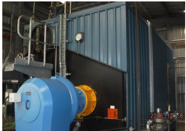
Figure 31. Biogas boiler
