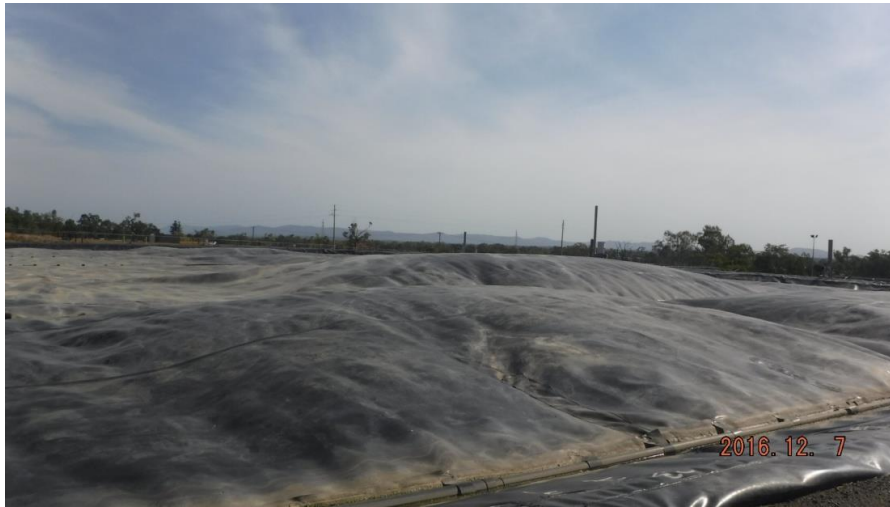
Figure 27. Biogas under the CAL1 cover at the Teys. Rockhampton WWTP
