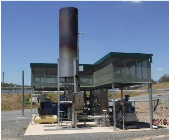
Figure 16. Biogas Flare
