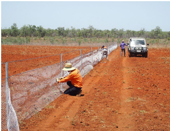
Applying mesh fencing to a fully prepared site at 'Spyglass'.
