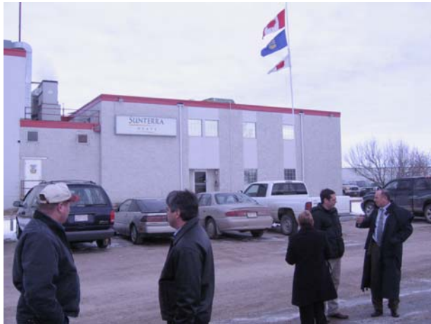
Sunterra Meats packing plant, Canada
