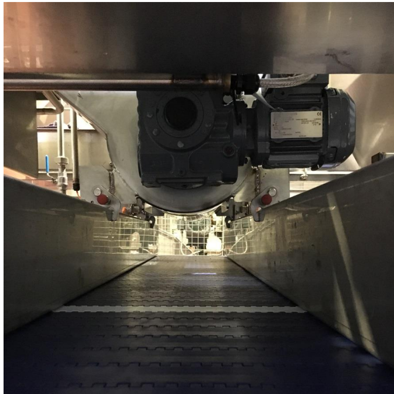
Figure 4: Auger discharges onto belt
