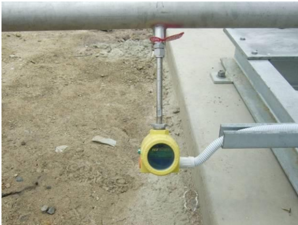
Photo 11: Inline FCI biogas flow meter
