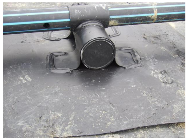
Photo 7: Sludge pipework weights
