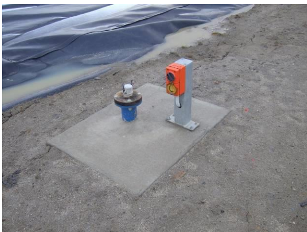
Photo 6: Sludge pipework upstand
