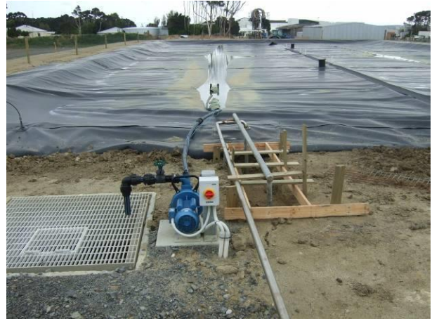
Photo 4: CAL showing stormwater removal
