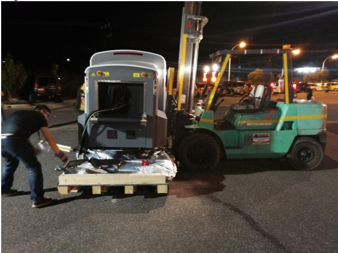
Image 1 installation of scanner
