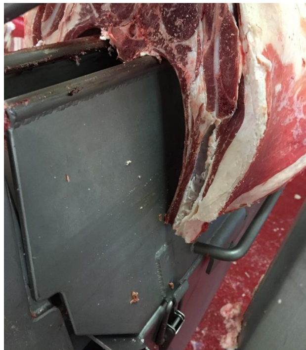
Figure 27: Gap at interface of loading station cover and product pusher chain cover is a snag point
