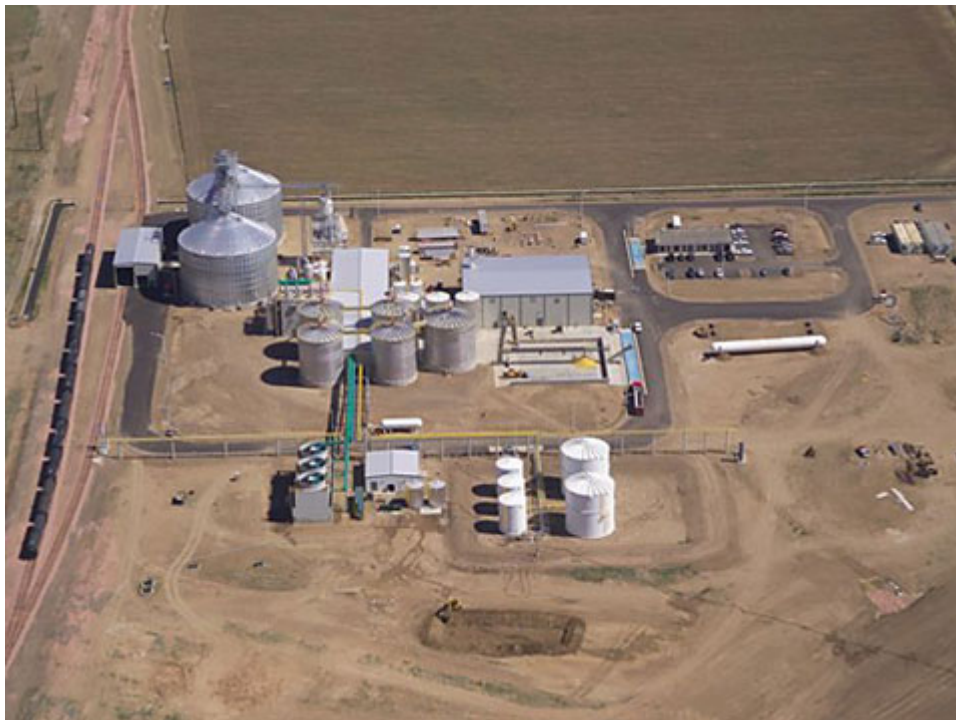
FIGURE 2 - TYPICAL GRAIN-BASED ETHANOL PLANT - FRONT RANGE ENERGY IN WINDSOR, COLORADO, 182 ML/YR (TAKEN FROM WWW.PACIFICETHANOL.NET )
