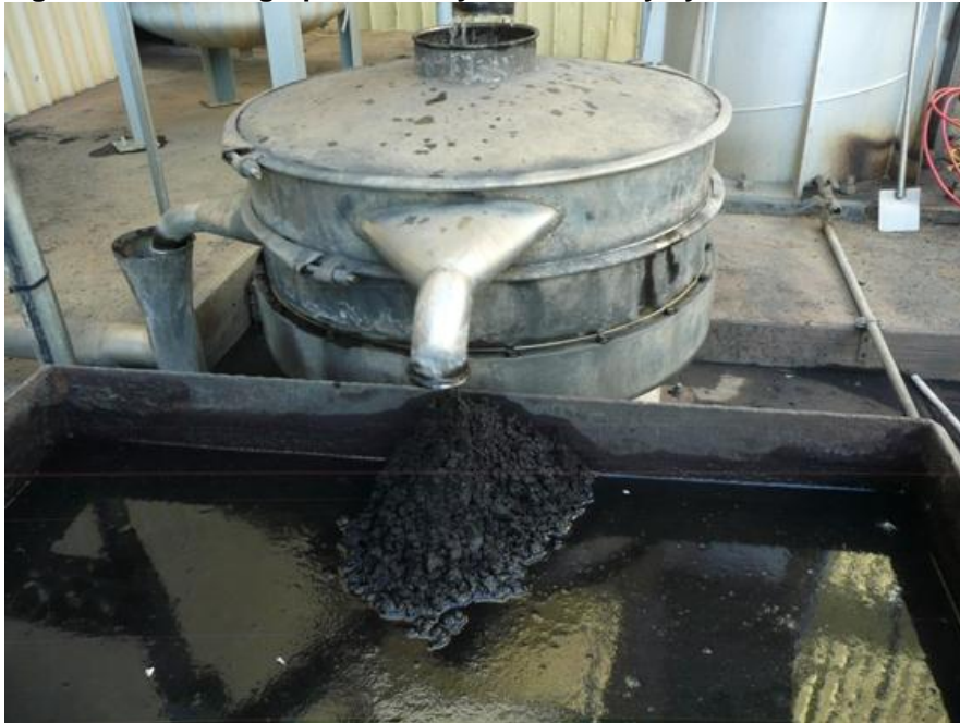
Figure 4.10: Photograph of wet fly ash recovery system
