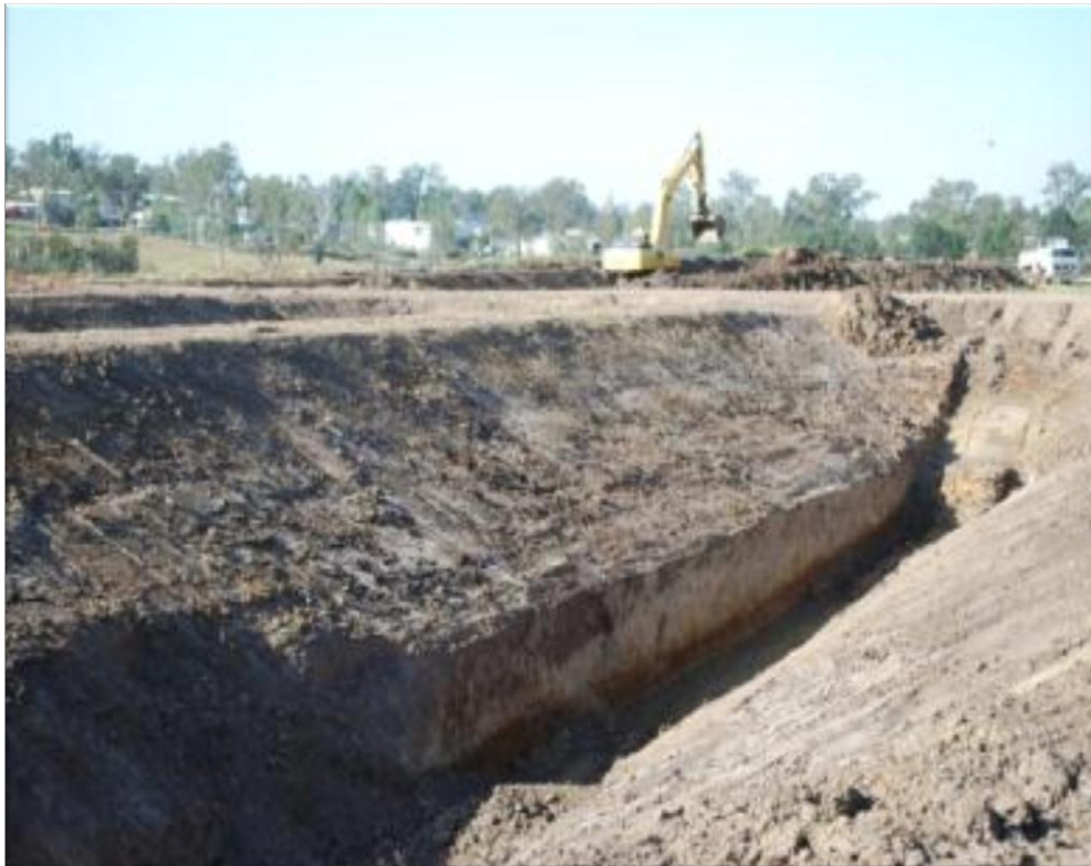
Figure 1.5: Pond D showing gravel bed of prior stream during construction
