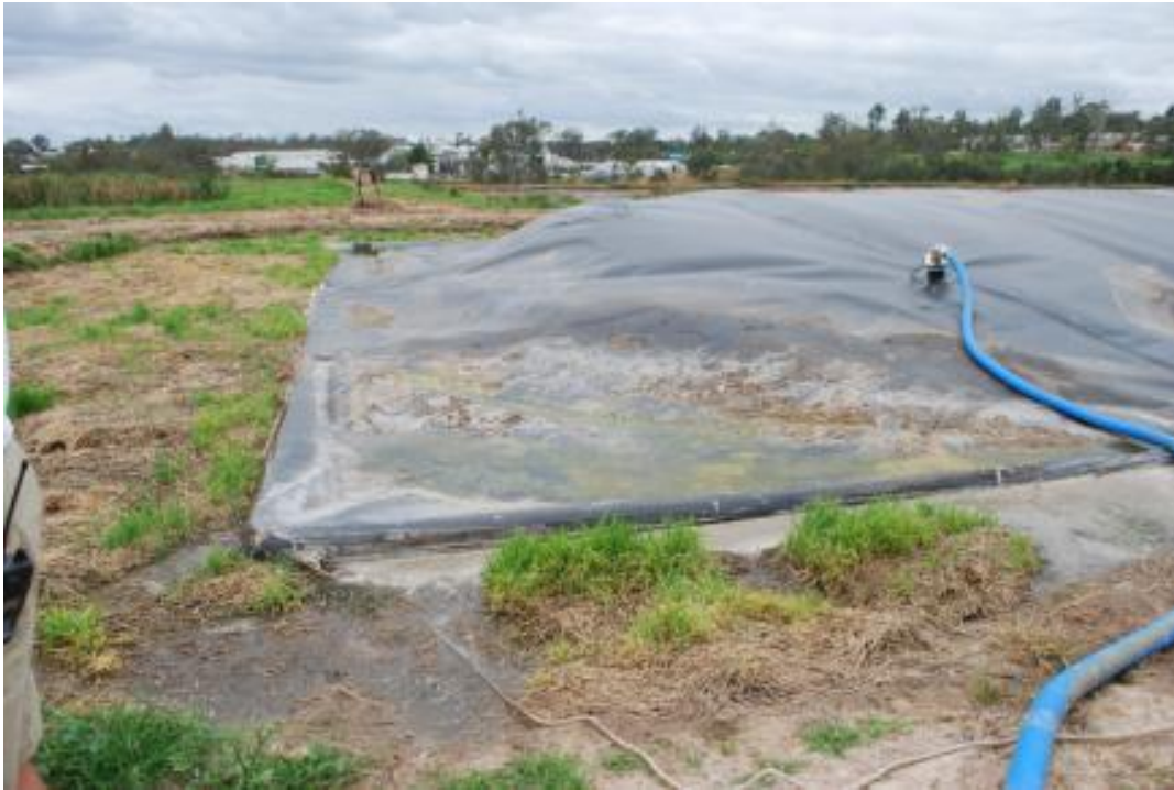
Figure 1.11: Interim arrangement for gas collection using 75mm flexible hose
