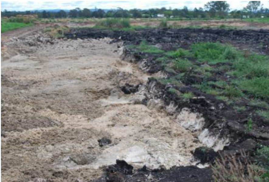
Figure 1.4: Desludging of Pond 1 and removal of crust in 2006
