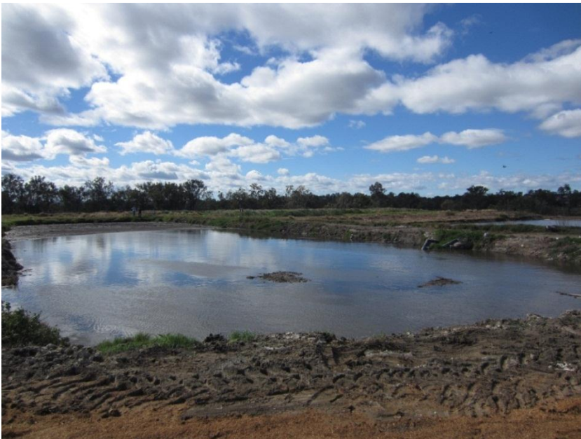
Figure 4.17. Desludging of pond A recently complete showing clean water awaiting re-commissioning of cover.
