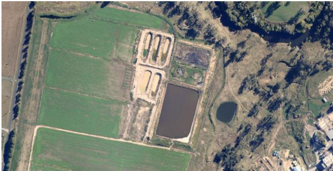
Figure 1.6: Aerial view of the ponds shortly after construction (source: http://www.nearmap.com/?ll=27.646008,152.739127&z=18&t=h&nmd=20100605 )
