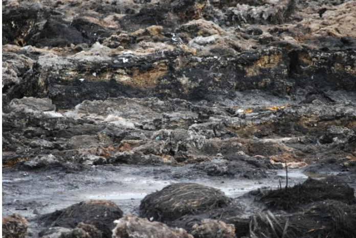
Figure 4.5a: Appearance of crust accumulation on pond A at the end of 2011 prior to desludging
