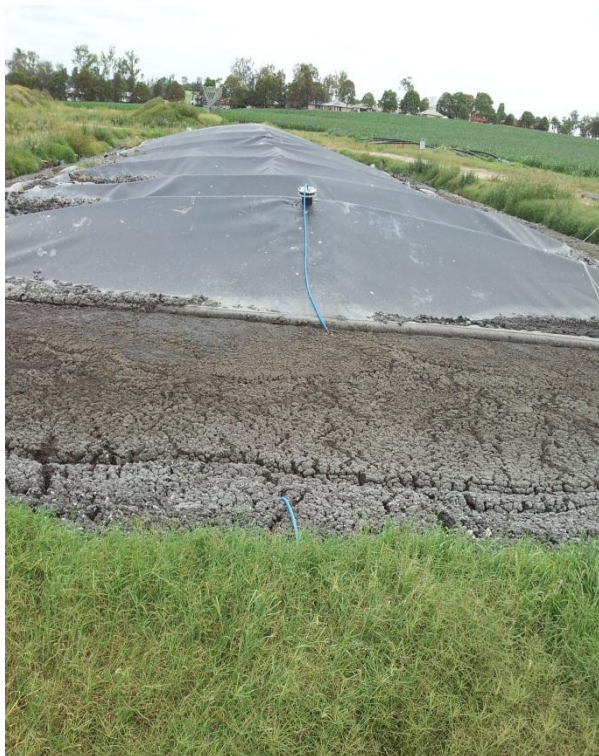
Figure 4.5b: HDPE cover on pond B showing the tube supplying the gas analyser with biogas from the pond. Note the presence of the thick crust
