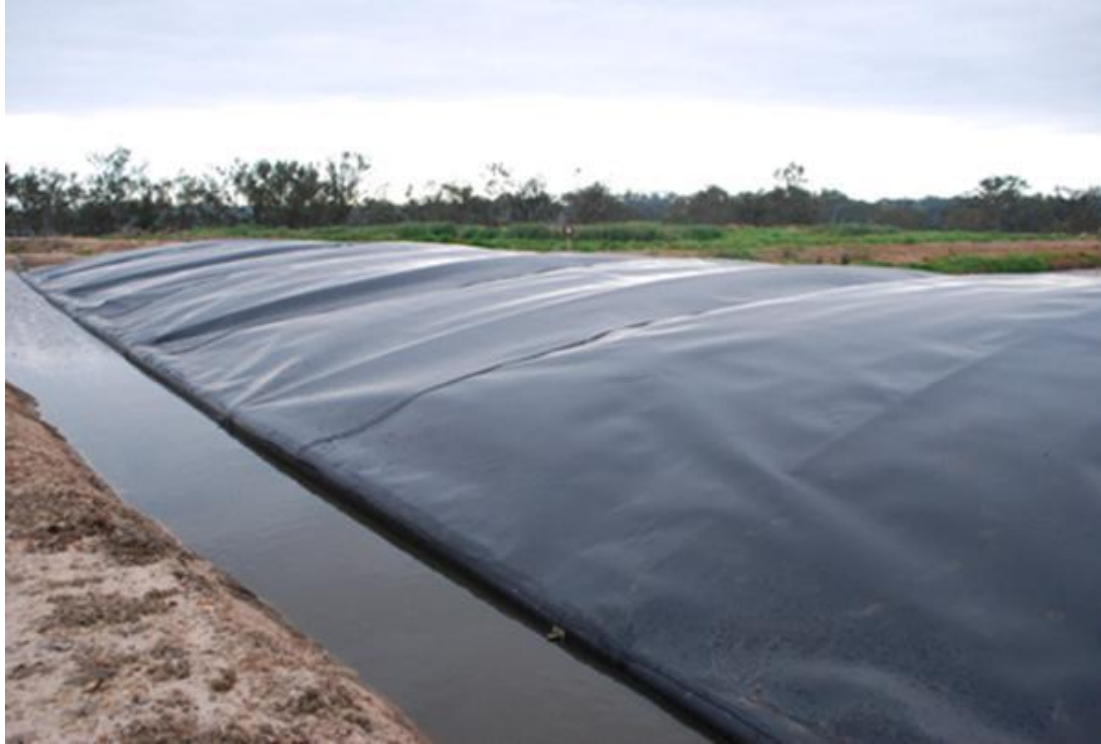
Figure 1.10: Installed cover on first pond, inflated with captured biogas.
