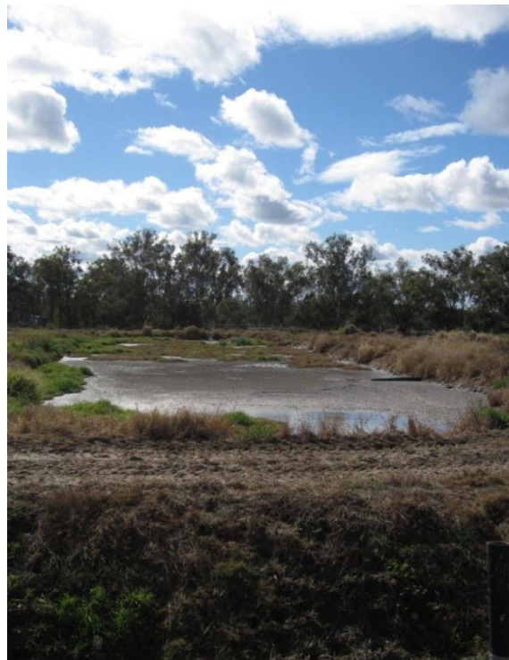
Figure 4.6: Relatively crust-free pond E. Straw was placed periodically on the pond to promote anaerobic conditions and reduce odour.
