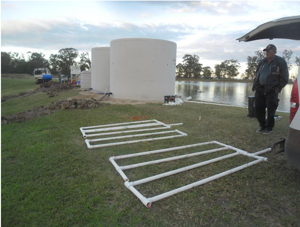
Figure 7: Internal arrangement of distribution pipe-work
