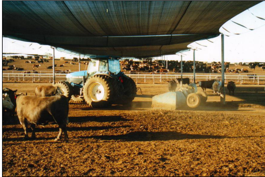
Figure 5. A shade cloth covered feedlot shade structure.
