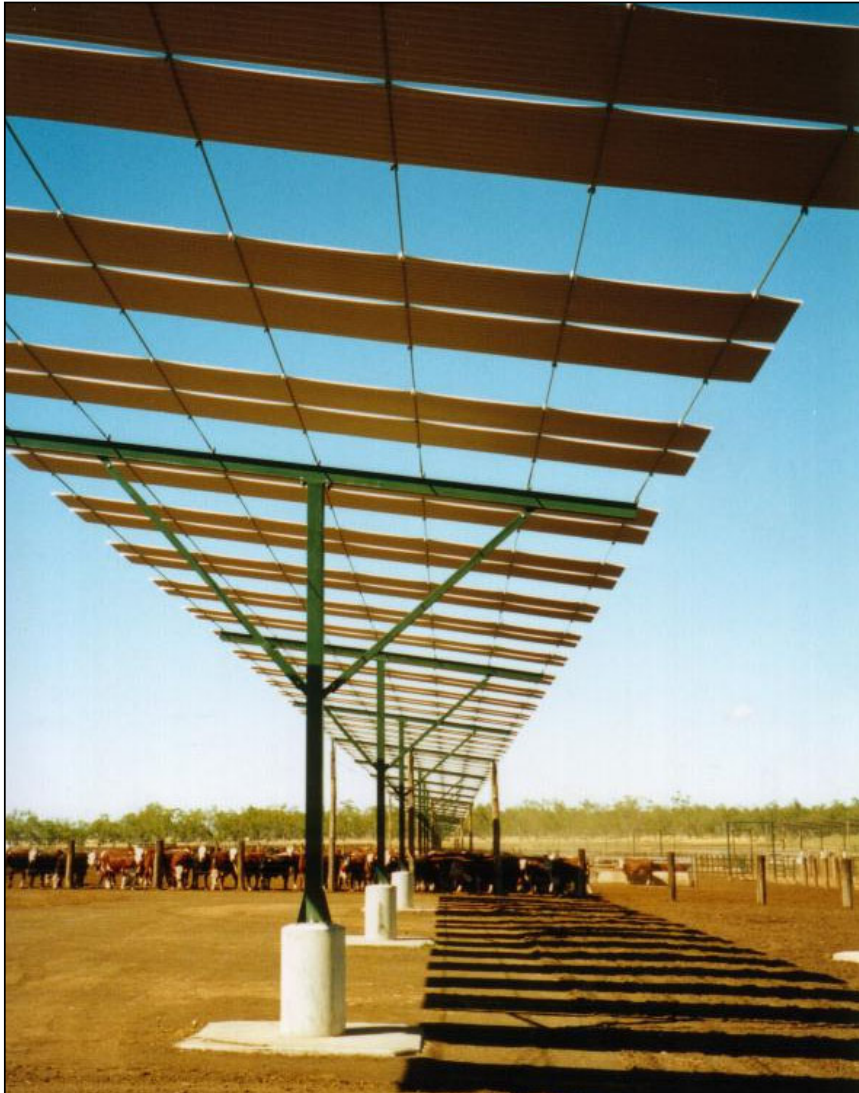
Figure 7. New shade structures constructed at Feedlot B.
