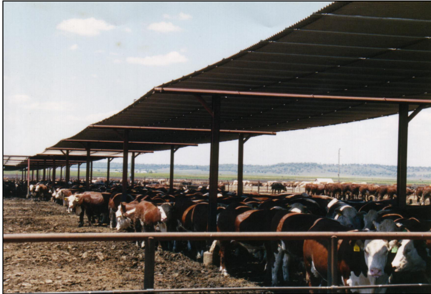
Figure 4. A sheet & cable feedlot shade structure with a variety of spatial configurations of sheeting.
