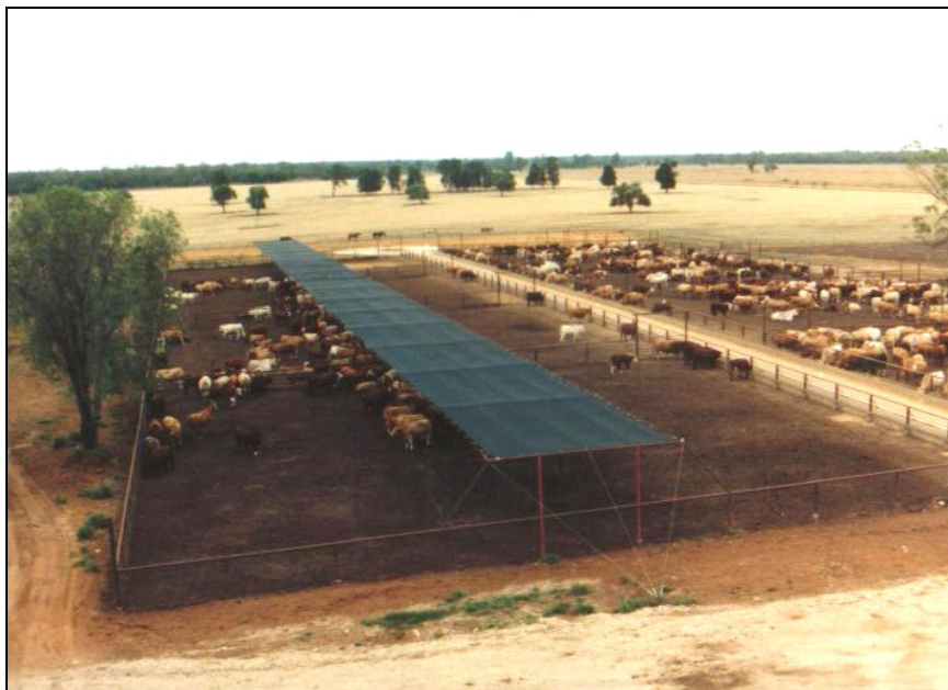
Figure 11. An effective current design of a shade structure utilised in Australia constructed from sloped shade cloth.
