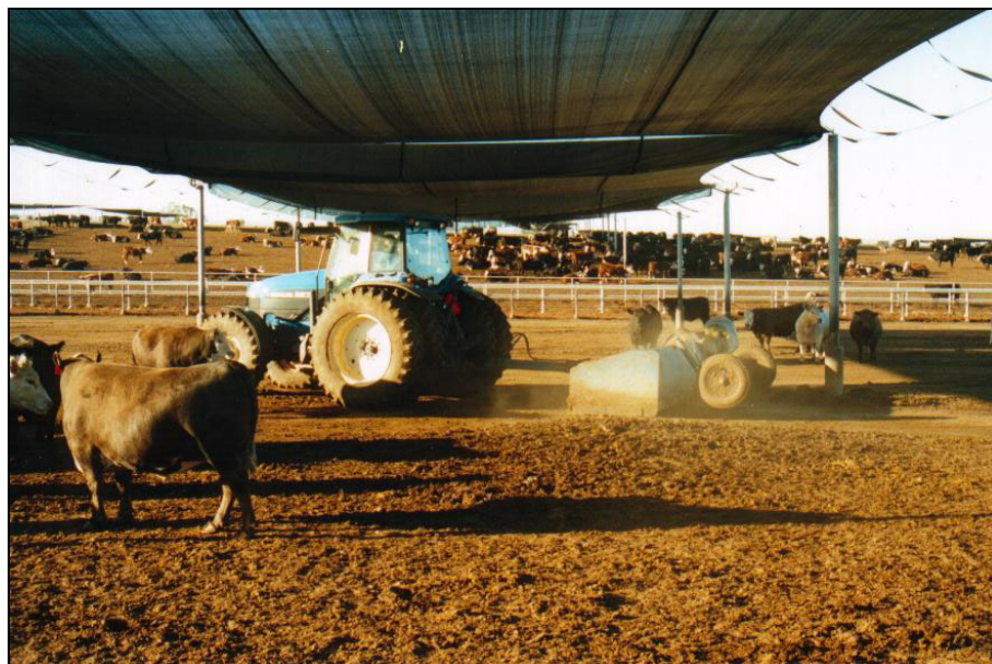
Figure 5. A shade cloth covered feedlot shade structure.
