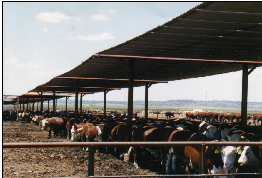
Figure 4. A sheet & cable feedlot shade structure with a variety of spatial configurations of sheeting.
