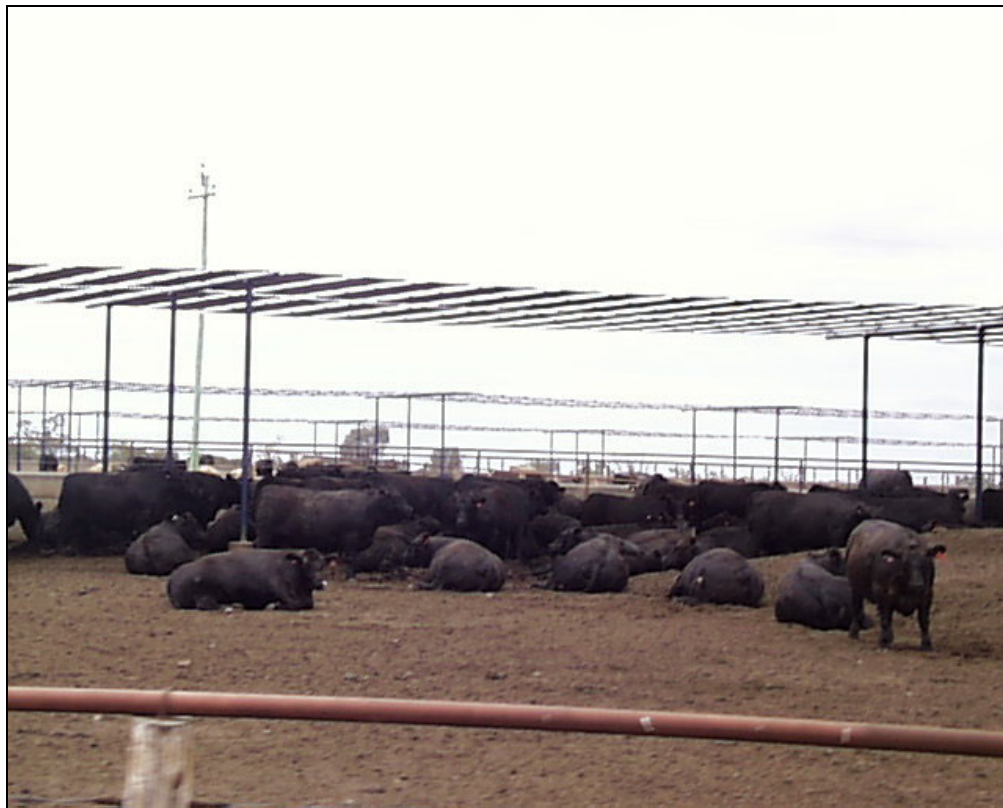
Figure 6. Shade structure at Feedlot A utilising corrugated iron sheeting.
