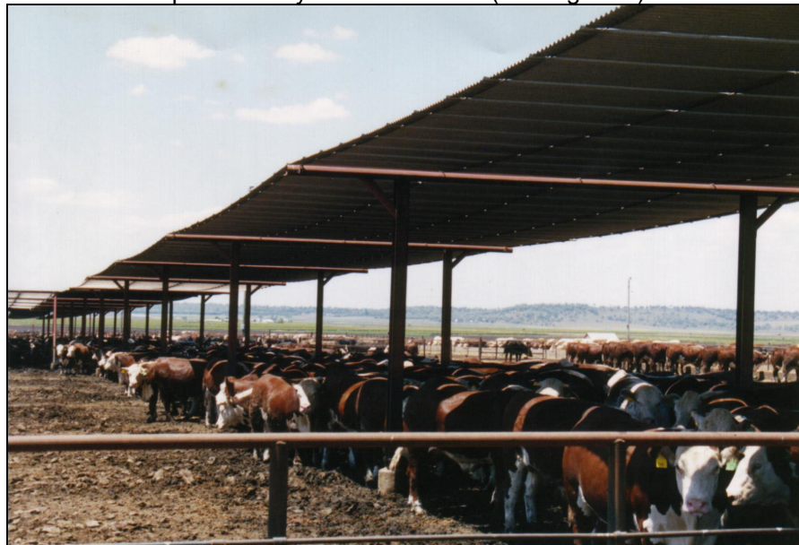
Figure 2. A sheet & cable feedlot shade structure with a variety of spatial configurations of sheeting.
