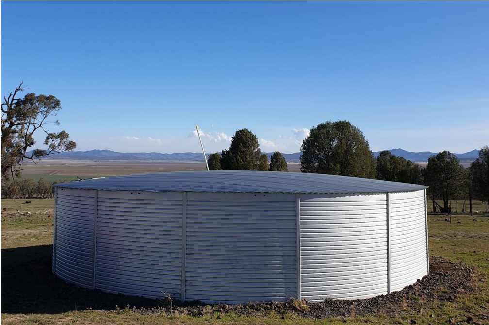
Figure 3. Water Tank at Windy Station
