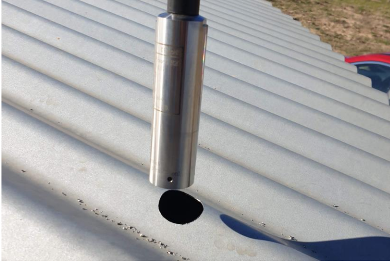
Figure 4. Hydrostatic pressure sensor installation.
