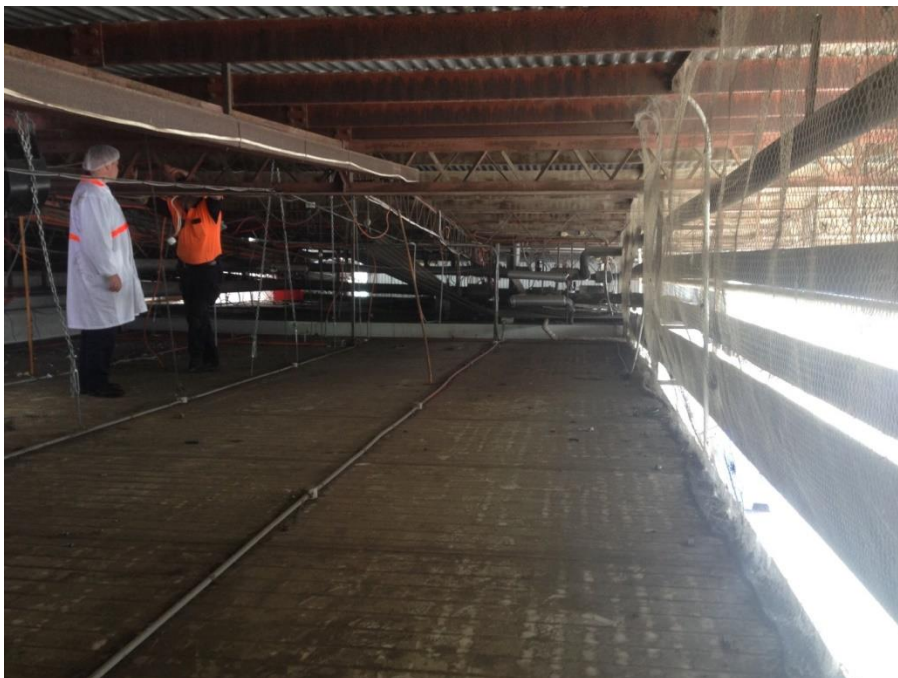
Fig. 2: Ceiling Cavity above Forequarter Machine Installation Room
