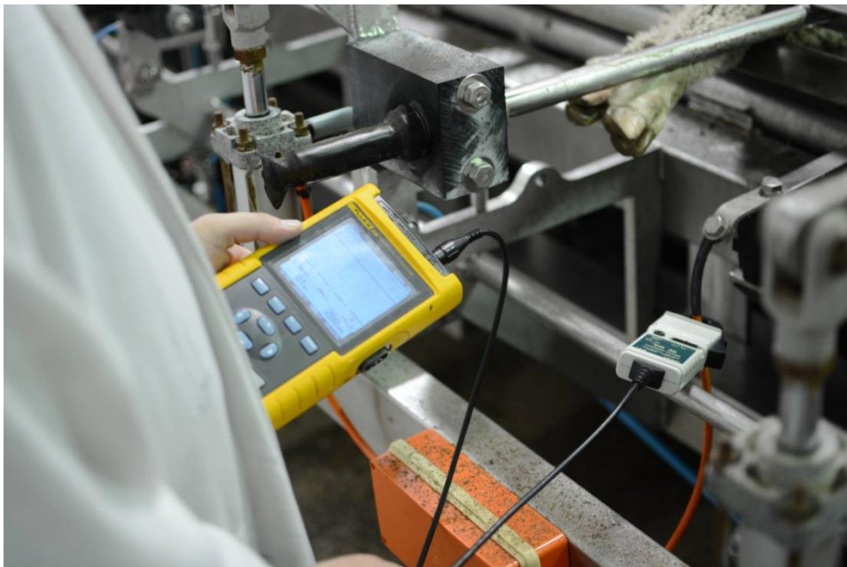
Photo 2: Current measurements being undertaken.
