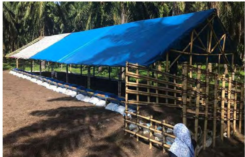
Cheaper ramps and sheds may be satisfactory for unloading small numbers of stock but may not endure with time and heavy use.
