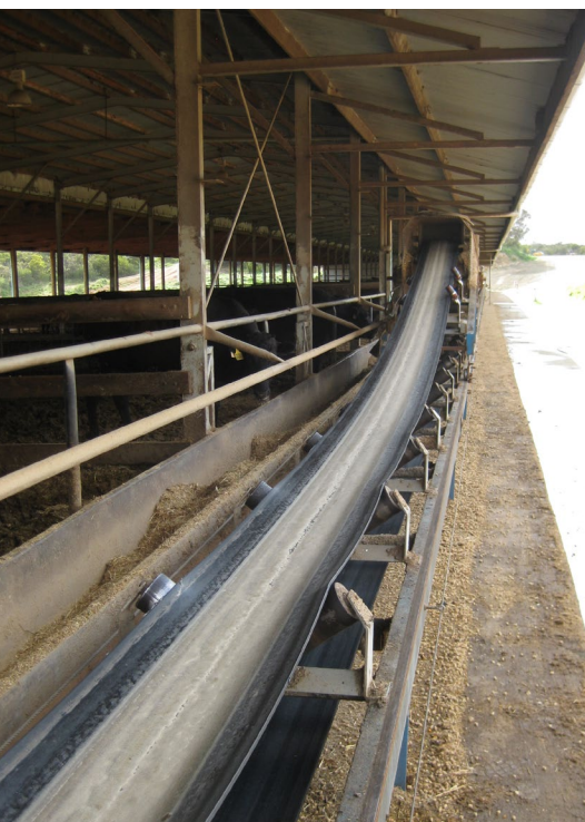
Single row housing with delivery of feed by gantry system running on fixed rails and connected to conveyor belt.
