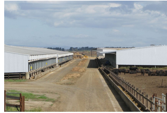
Roof water collection system
