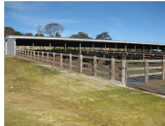
Partially covered single row housing system
