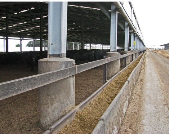
Single row gabled roof system with uncovered feed bunk
