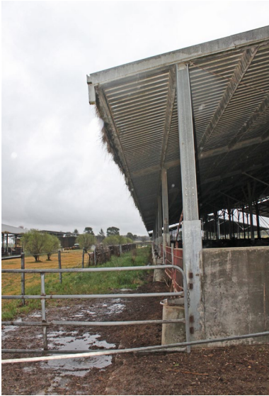
Half-covered cattle lane running length of shed – roof is guttered to prevent runoff directly into cattle lane.
