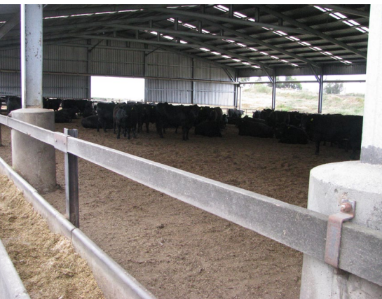
Gable, trussed roof with sheeted end wall
