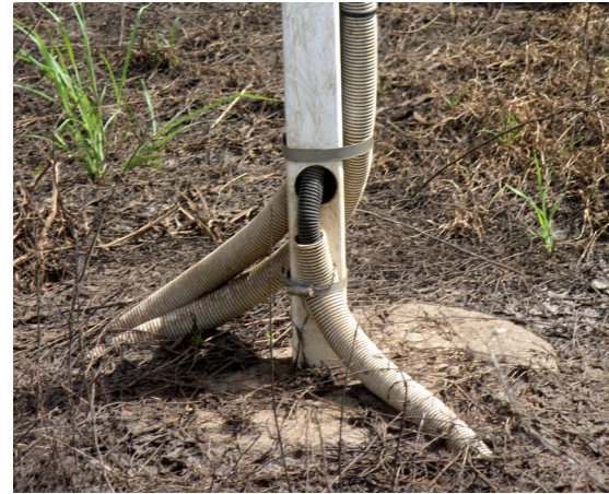
All cables to and from the AWS need to be protected from damage by machinery and animals. Cockatoos and rodents chewing on exposed cables lead to loss of data and expensive repairs.
