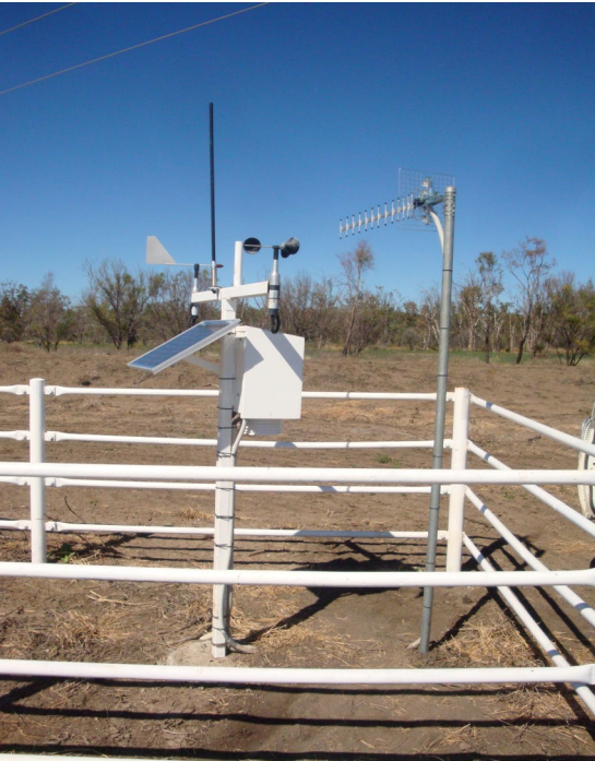
Typical 2 m solar-powered AWS with remote access.
