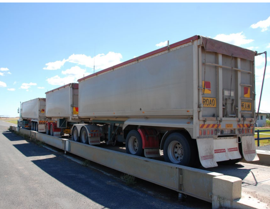
A multiple deck weighbridge allows the truck to be weighed in a single measurement.
