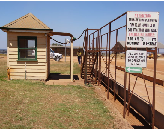
Weighbridge with good signage and a long sampling platform, allowing load to be inspected or sampled without repositioning the trailer.
