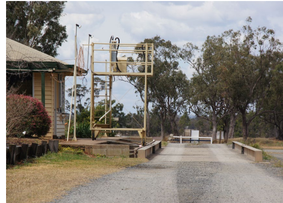
The length of approach will depend on the overall length of the weighbridge. Note proximity to the site office.
