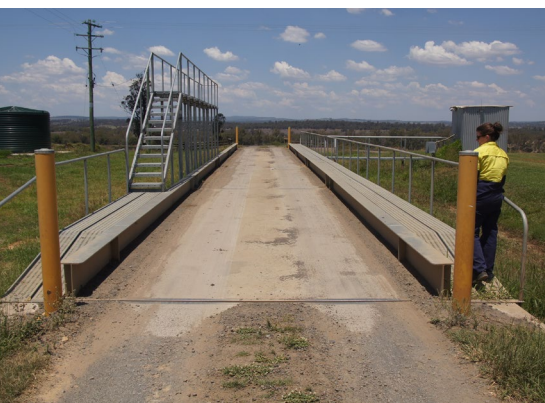
Boldly painted bollards placed at the entry and exit guide the truck driver and protect the weighbridge sides.
