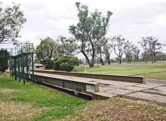
Above-ground truck weighbridge with commodity sampling platform.
