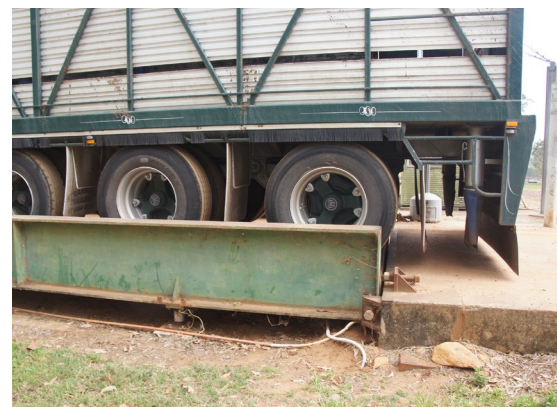
This weighbridge platform is too short for weighing prime mover and trailer together.
