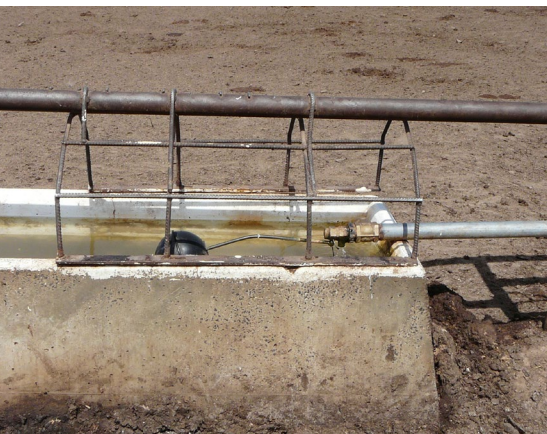
Steel cage to protect float
