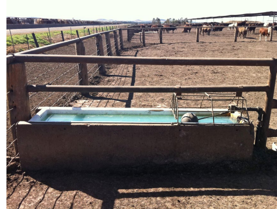
Fibreglass insert in a trough (Position D).
