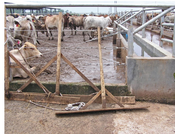
A water trough placed across the bottom fence will prevent proper pen drainage – a poor design choice.
