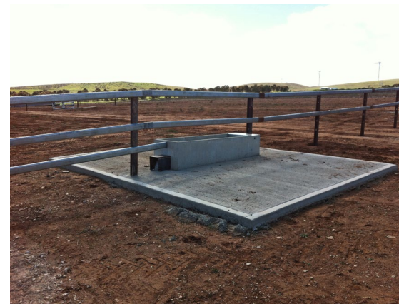
Aprons allow cattle to access to the trough under all weather conditions and allow access for cleaning (Position A).
