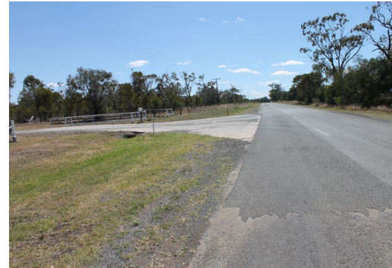
Concrete pavement on feedlot access road to prevent road damage caused by heavy vehicle traffic at turn-in and turn-out
