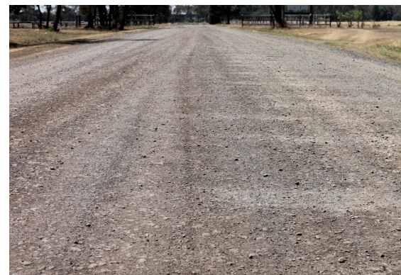
Unsealed road with a well-maintained and shaped crown, shoulder and v-drains
