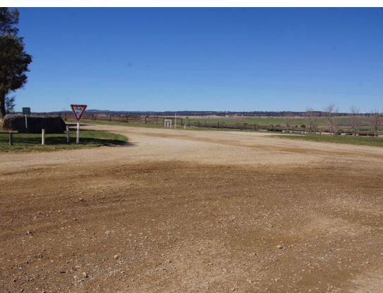
Staggered T-intersections have fewer conflict points than 4-way intersections.
