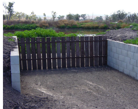
A single row vertical timber weir, with no overtopping freeboard
