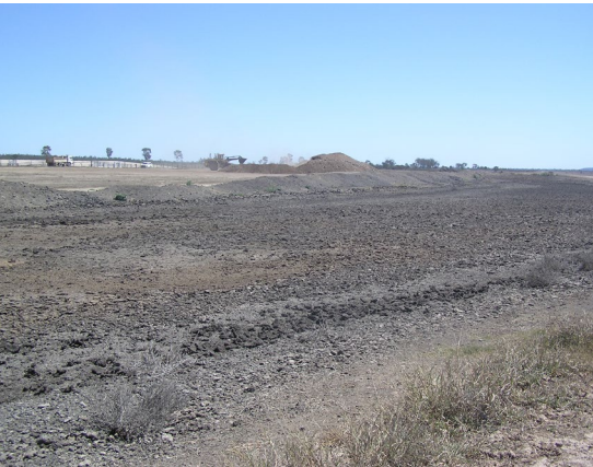
Sediment basin effectively retaining sediment and draining to bed level, allowing deposited solids to dry.
