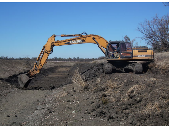
The excavator must have suitable reach and digging depth.
