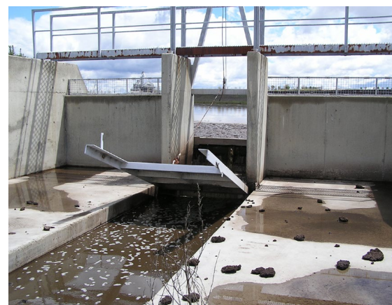
A drop weir structure on a sedimentation basin relies on human intervention for use. Thus the operation of the system can be stalled if workers cannot reach the sedimentation system as during flooding.
