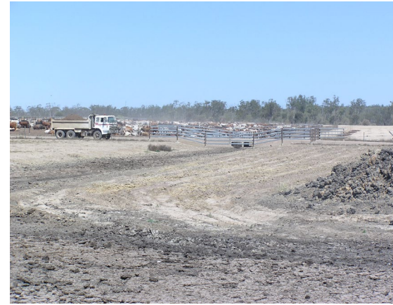
A view upstream of the sedimentation system showing the drainage line from the pens to the sedimentation system. The drains run under an on-site roadway, through a concrete culvert that permits the uninterrupted flow of effluent to the sedimentation system.
