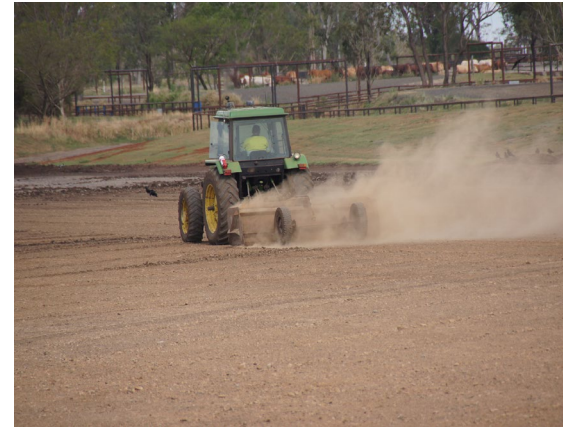
Maintenance of the base of the sedimentation system with a box scraper. Dual sedimentation structures before the holding pond will allow one to be de-silted while runoff is diverted to the other.
