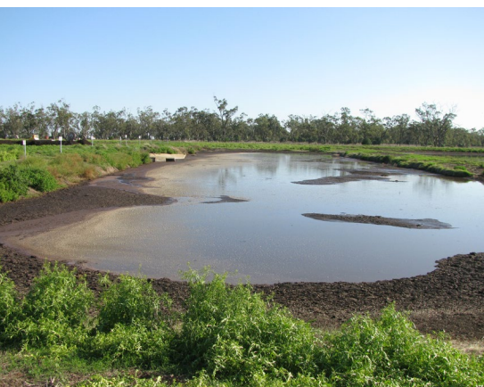
A sedimentation pond (5 m deep) that stays full of liquid. This pond has an inlet weir for incoming sediment and effluent runoff, and an outlet weir to a shallow, large surface area evaporation basin.
