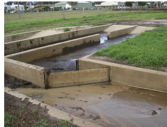
Effluent can be diverted into one side of the basin so that the other side can dry out and sediment be removed.
