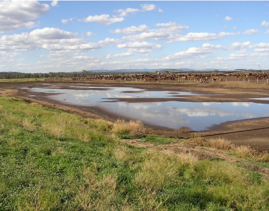
A large shallow sedimentation basin drying out after storm runoff
