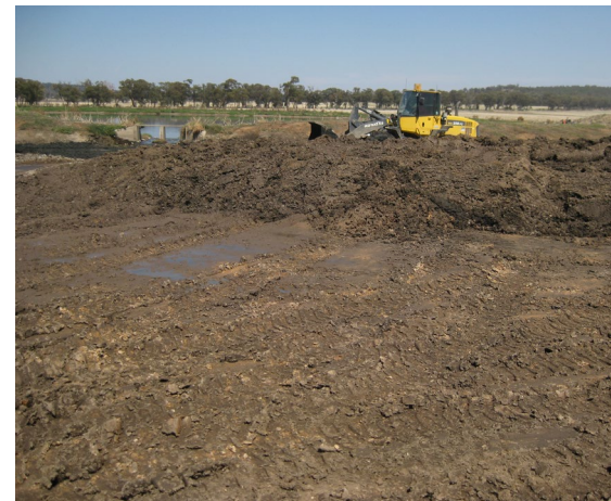
Cleaning out a sedimentation basin in relatively wet conditions is not desirable as wet sludge is difficult to handle, store and will not dry out.
