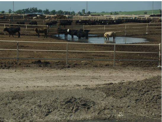
Pen to pen drainage is a poor design.
