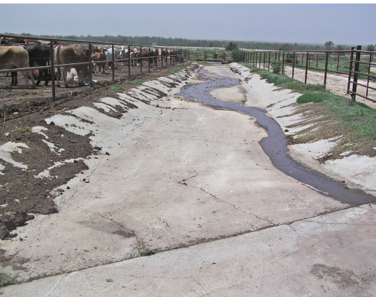
Concrete drains can be used in steep drain sections to prevent erosion. However, the drain must be wide enough to allow access by cleaning equipment.
