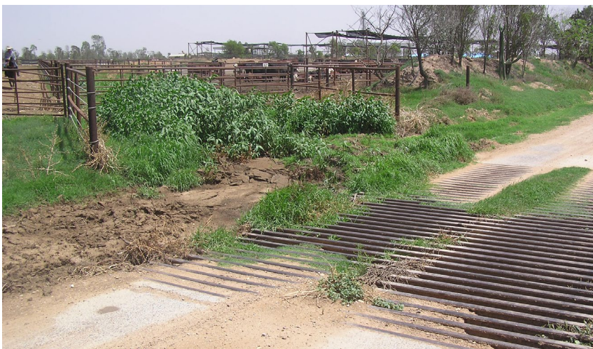
Grid culvert drain crossing makes it difficult to clean under the grid.
