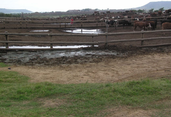
Drains should not be formed in the middle of the pens as they promote pen to pen drainage. Note how the lower rail on the fence blocks drainage.
