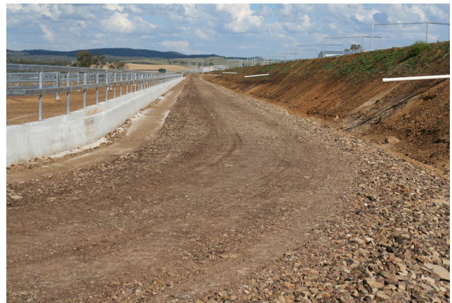
Feed roads need 2–3% slope for adequate drainage.
