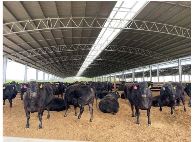
Photograph 25: Ridge vent in convex roof
