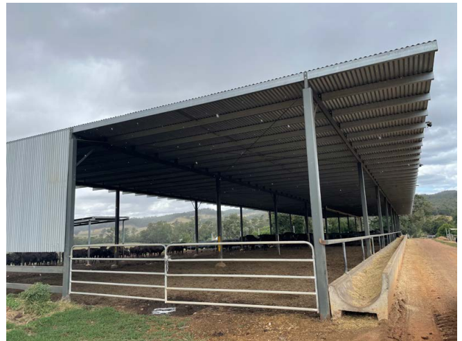
Photograph 2: Monoslope roof design
