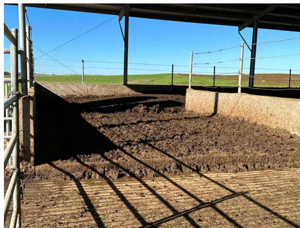
Ramp from feeding area to compost bedded pack area
