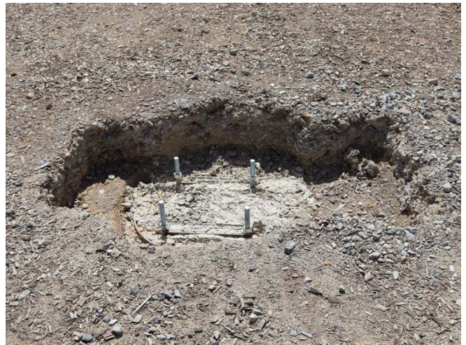
Photograph 17: Concrete pier footing with anchor bolts
