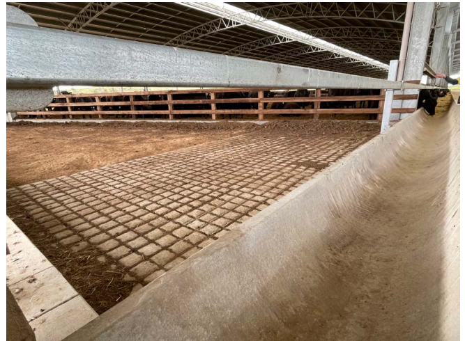
Photograph 34: Non slip stamped concrete feed bunk apron
