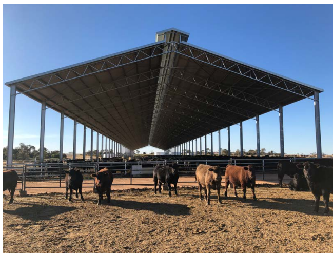
Photograph 24: Gable roof design with ridge ventilation
