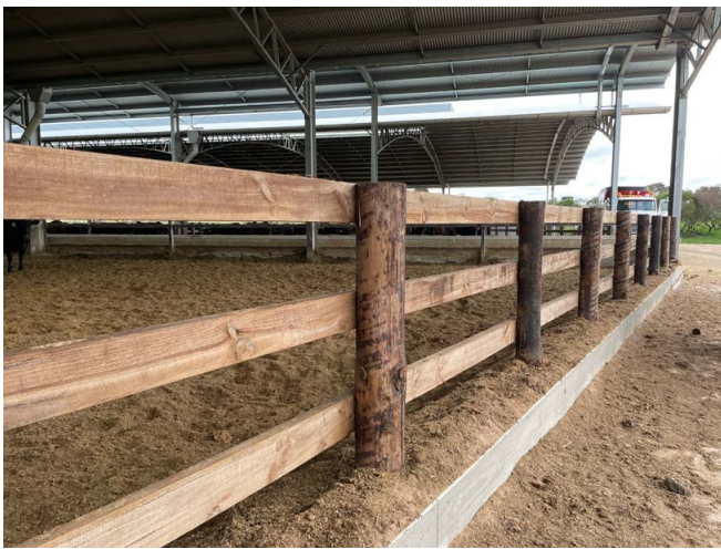
Photograph 47: A nib wall along the fenceline will help to keep bedding inside the pen
