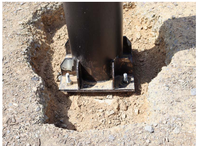
Photograph 19: Bored concrete pier footing set below pen surface
