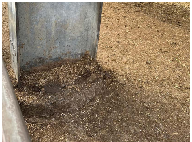
Photograph 18: Bored concrete pier footing set above pen surface
