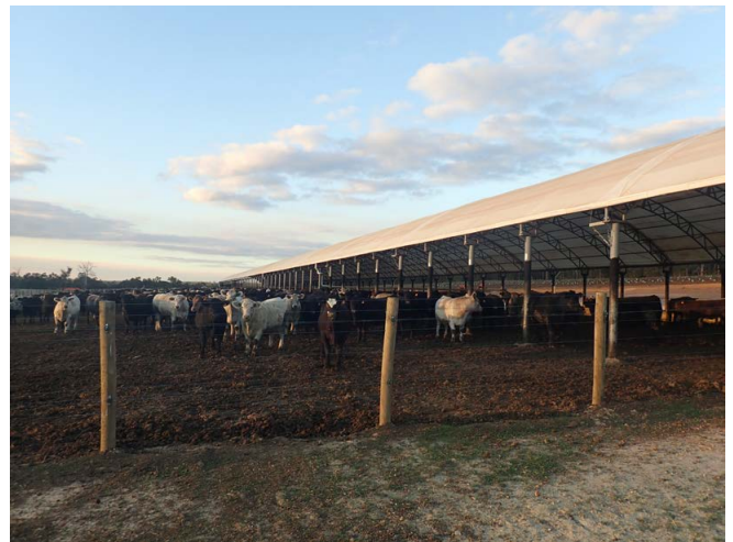
Photograph 6: Hoop structure convex roof
