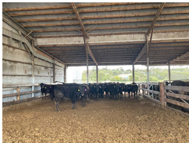
Photograph 33: Cladded end wall on covered housing system
