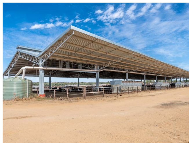
Photograph 42: Self-feeders need sufficient roof height for filling
