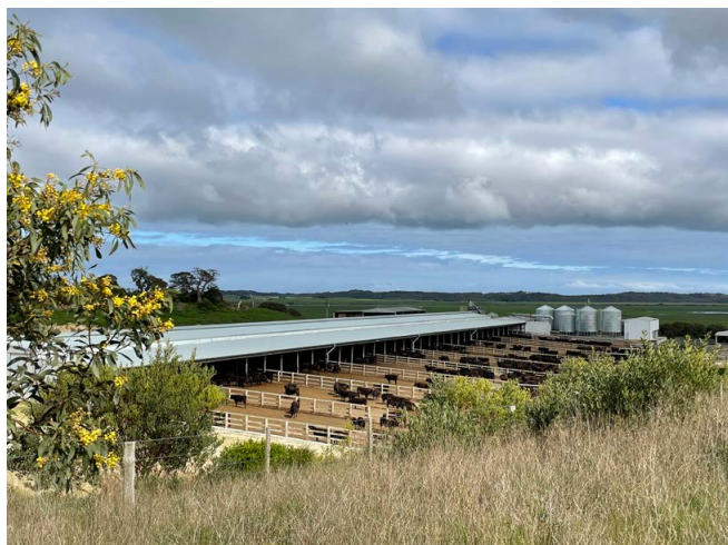
Photograph 7: Partial pen covering is an effective option for retrofits
