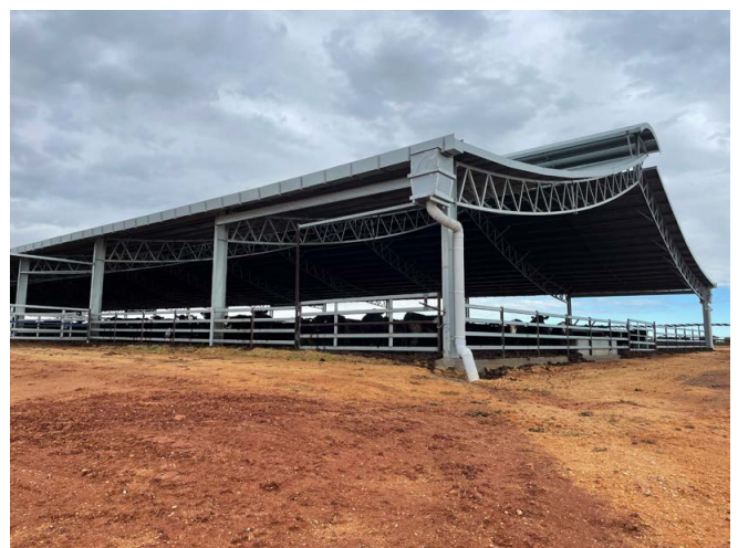
Photograph 26: Covered ridge vent on a concave roof
