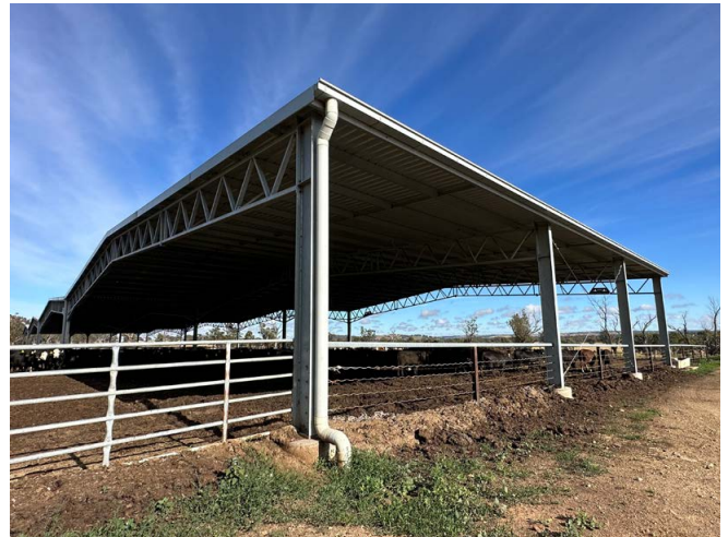
Photograph 37: Cattle rail and curly cables effectively contain cattle
