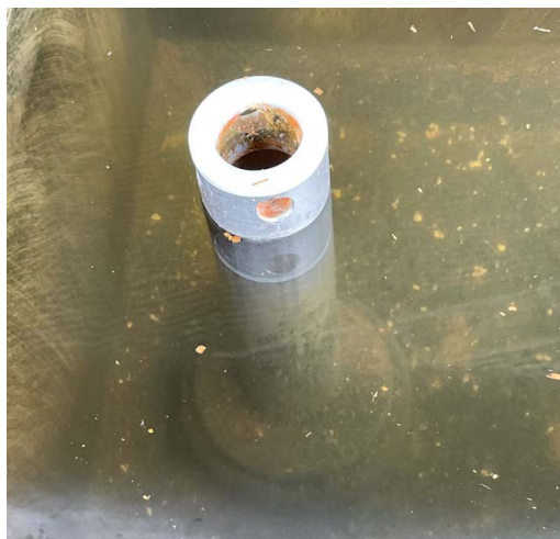
Photograph 46: Water trough overflow pipe
