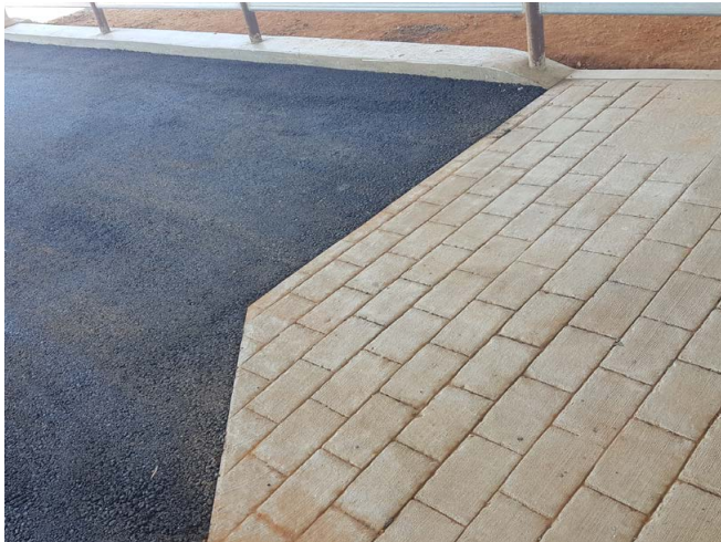
Photograph 35: Asphalt surface and stamped concrete water trough apron
