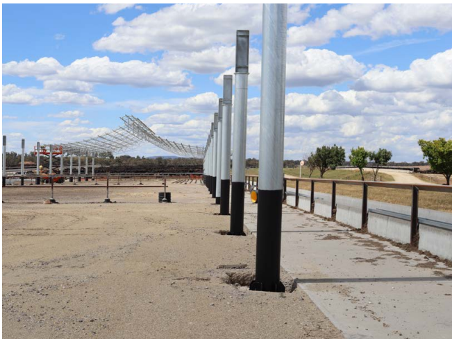
Photograph 20b: Circular hollow section
