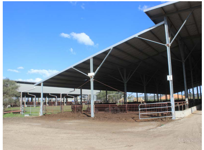
Photograph 21: Building support columns – Cold roll formed
