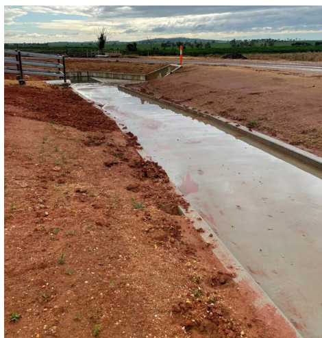
Photograph 45: Concrete catch drain
