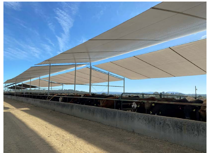
Photograph 29: Waterproof fabric used as partial pen cover
