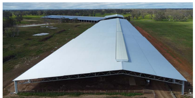
Photograph 3: Covered housing system with asymmetrical gable roof and ridge ventilation retrofitted over existing feedlot pens
