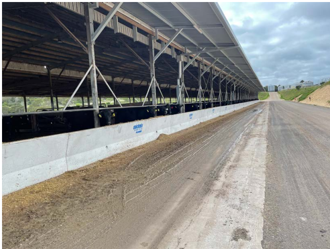
Photograph 13: Partly covered concrete feed alley
