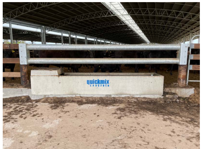
Photograph 36: Water trough surrounded by concrete apron
