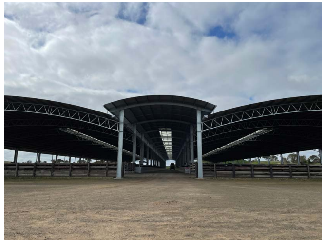
Photograph 5: Convex roof profile with truss
