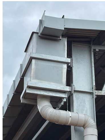
Photograph 32: Gutter and downpipe rain head system
