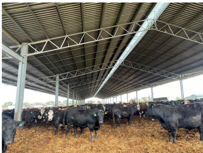
Photograph 30: Clear ridge vent cap in roof
