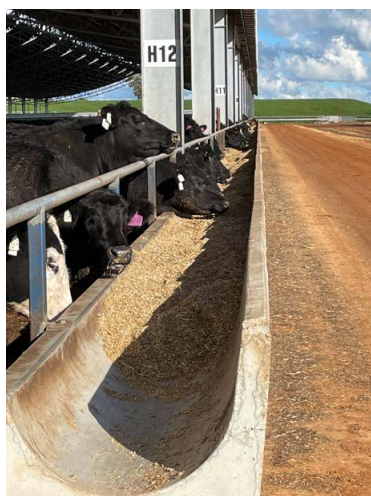
Photograph 41: Precast concrete feed bunk
