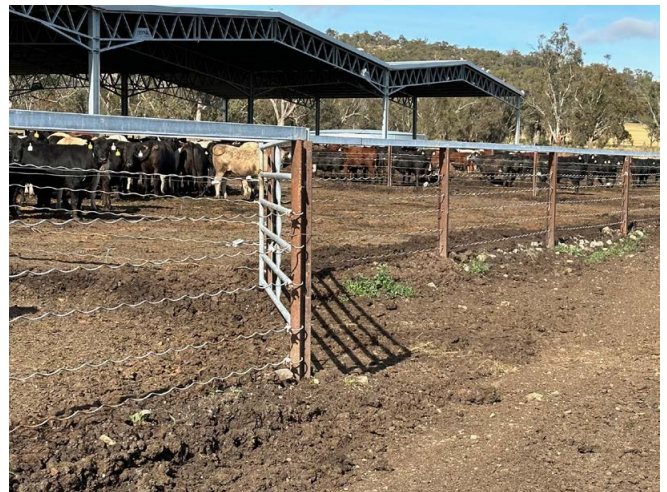
Photograph 39: Herringbone gate arrangement on cattle lane
