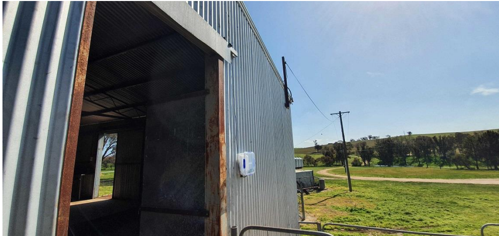
Figure 4 Temporary gateway installed on side of local shed on Romani property.
