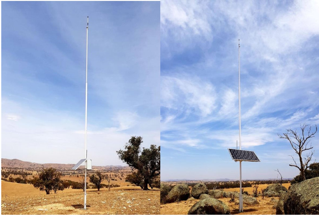
Figure 3: Redbank gateway installation photos
